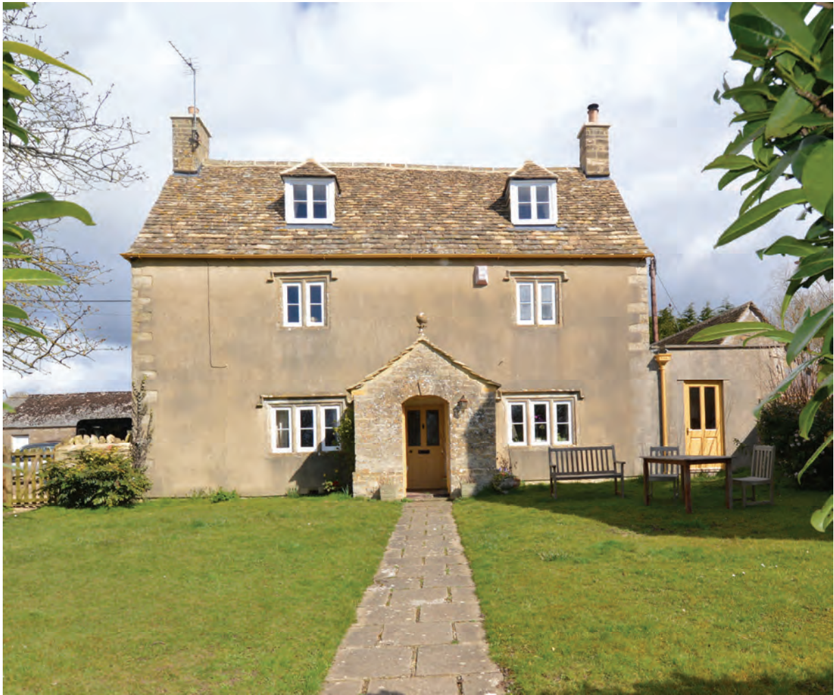
Fig 6. The farmhouse front elevation with the farm buildings visible behind.
