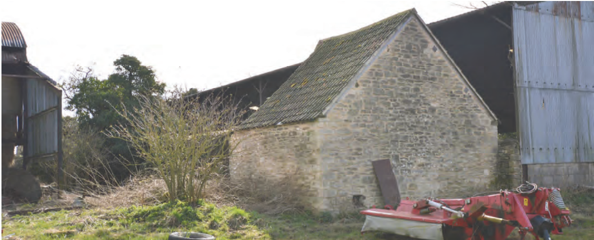
Fig 19. The restored free-standing barn in the north yard to the east of the access with its adjacent covered yard.
