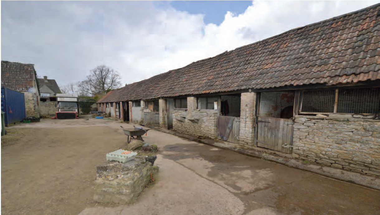
Fig 16. The north range looking west with Pond Cottage just visible beyond the site boundary in the distance. The stable cross wing of the south range is on the left. The nearer section of the north range has stone rather than brick piers and is slightly later in date, and is currently used as stabling.
