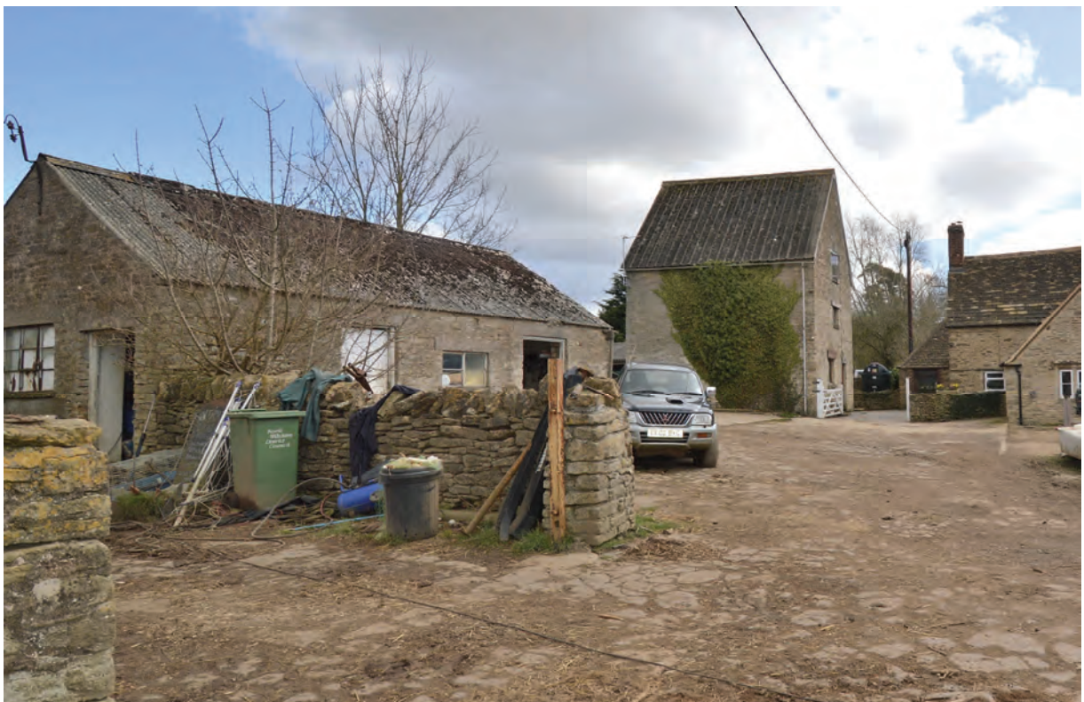
Fig 15. The altered outbuilding at the east end of the south range, with the farmhouse just visible on the right.
