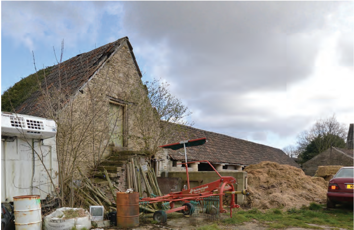
Fig 14. The south gable of the attached stable and hayloft showing the tallet steps and door.
