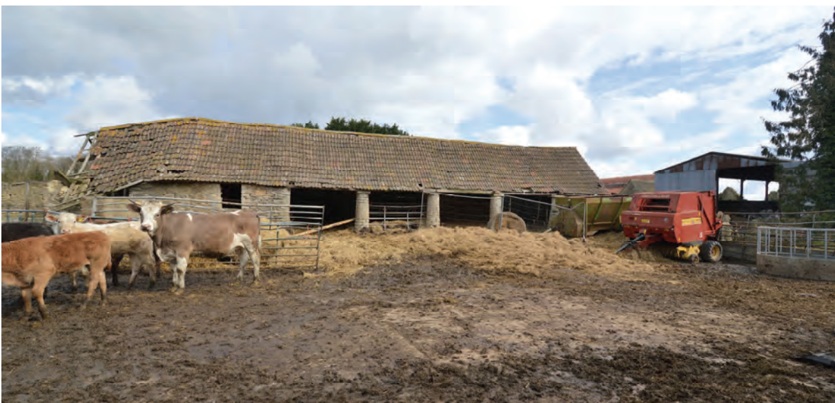
Fig 18. The partly collapsed barn on the north side of the north yard. Originally an L-shape, the return section survives only as sections of ruined structures.
