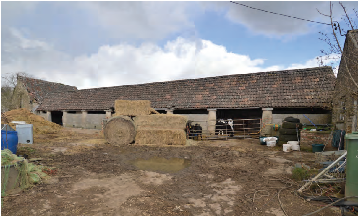
Fig 13, The south range with the stable cross wing at its western end. To the right is the gable elevation of the much-altered store.
