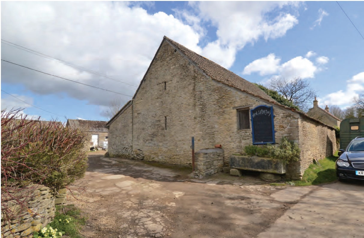
Fig 11, The main barn showing the full length southern lean-to and the western access into the farmyard.
