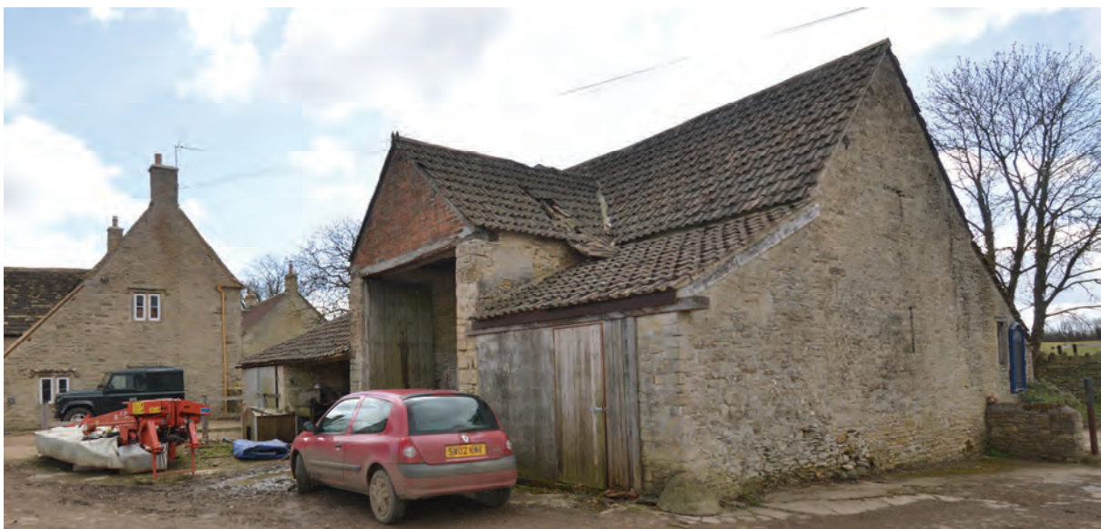
Fig 10, The main barn with its northern formerly open sided lean-tos on either side of the midstrey.
