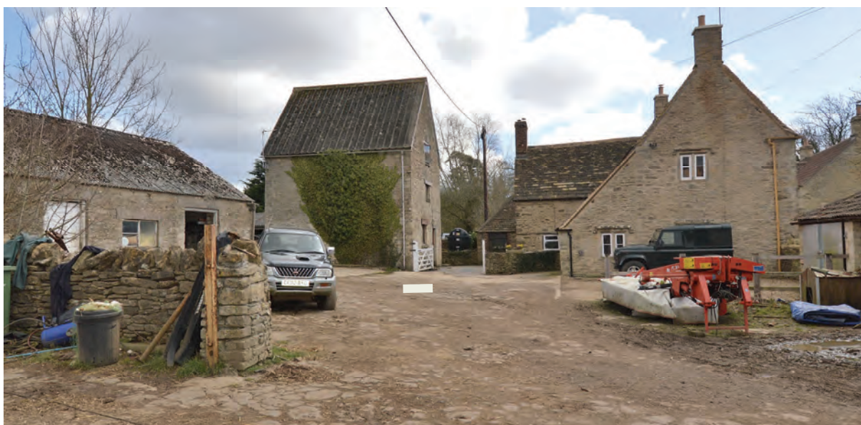
Fig 8. The tall outbuilding to the north of the farmhouse, with the adjacent much altered single storey outbuilding, define the north side of this farmyard. Behind the farmhouse is the hipped roof of a second single storey range perhaps originally a dairy or brew house now converted to residential accommodation.
