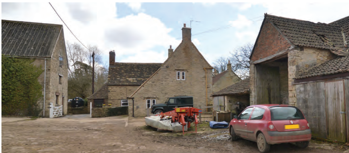
Fig 7. The farmhouse with its one and half storey north wing, seen behind the north lean-to with its cat-slide roof. Behind the north wing is the hipped roof of a single storey outbuilding and on the left is a tall free-standing building. The change in masonry above its first floor window shows where a further storey has been added.
