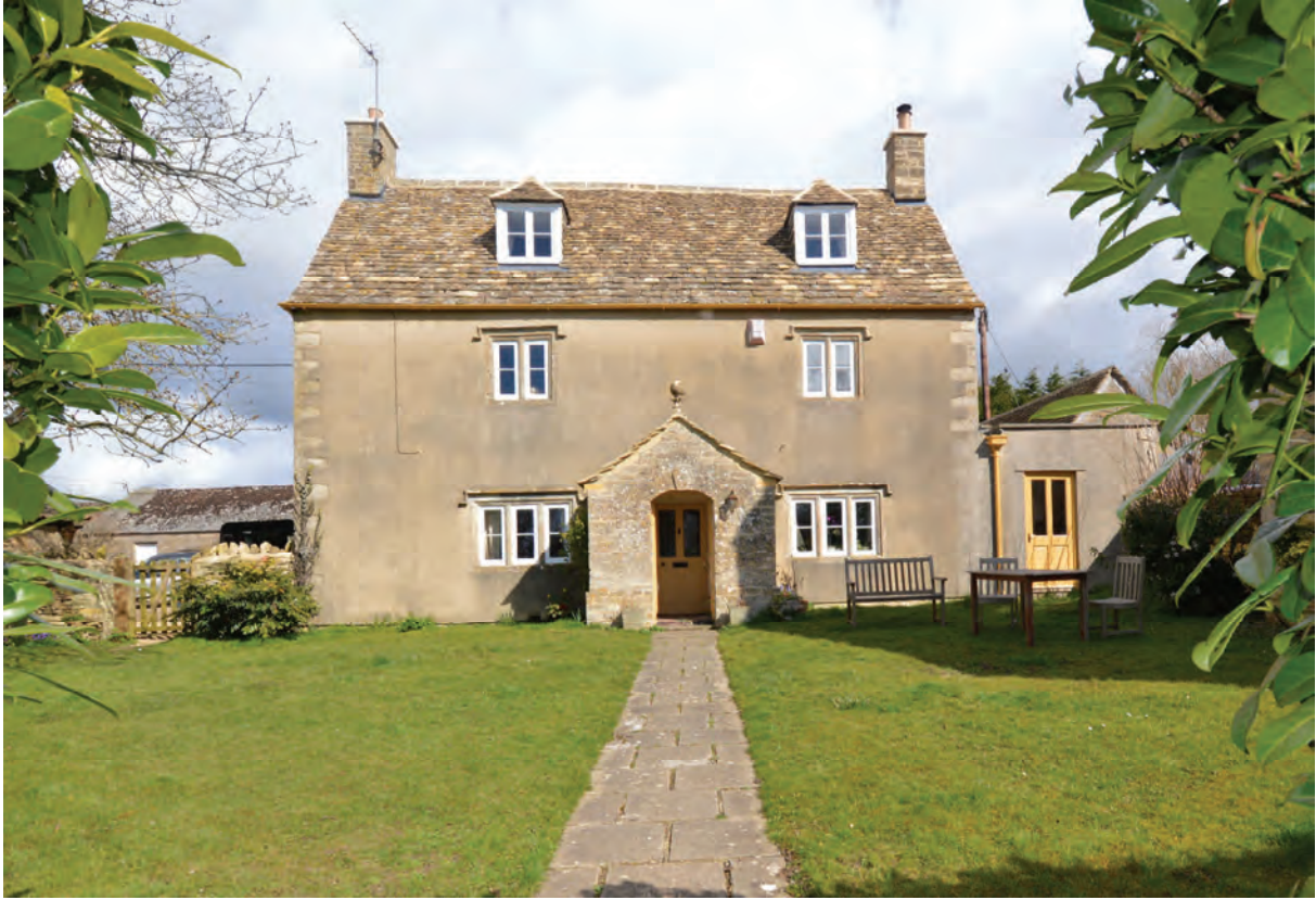
Fig 3, The principal south elevation of the farm house with the adjacent barns visible behind on either side.
