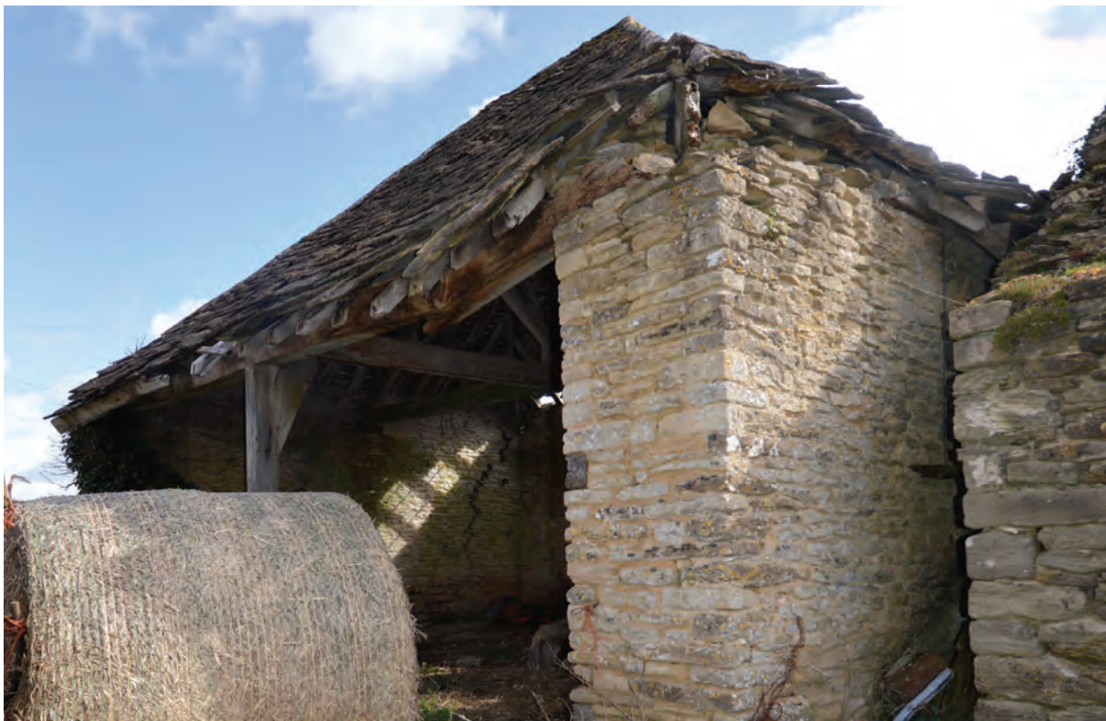
Fig 20. The roof within the hipped free-standing open-sided barn with jowled posts and king post trusses.
