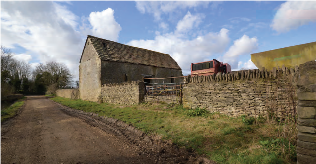
Fig 17. The north barn with enclosed yards to either side.
