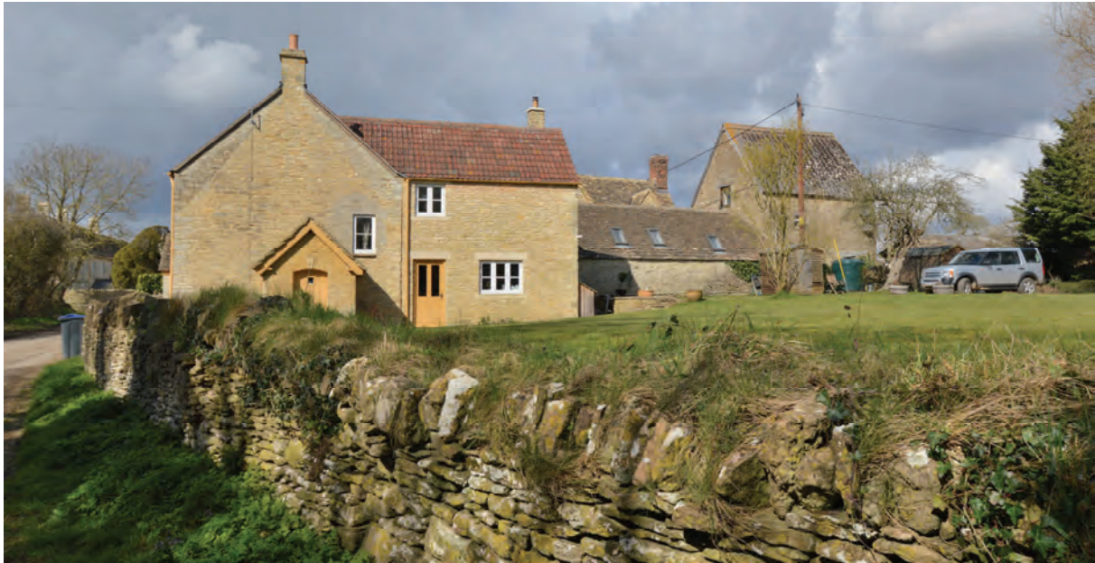
Fig 9, Townfield cottages with their well detailed but large modern rear extension and historic east gable porch.
