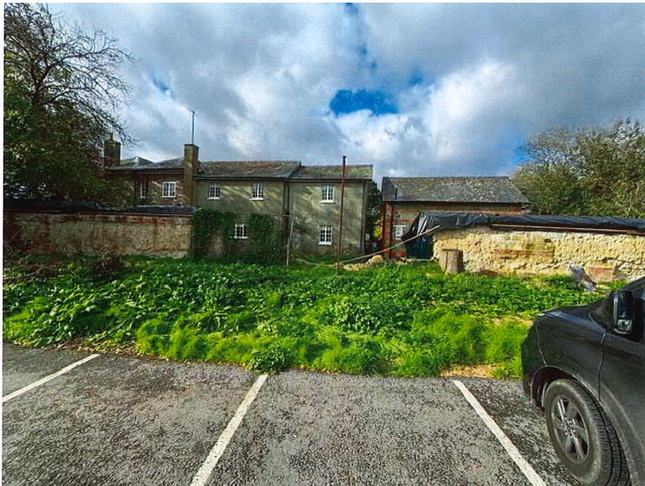
BOUNDARY WALL, THE BRADFORD INN, BRADFORD ST. MARTIN
