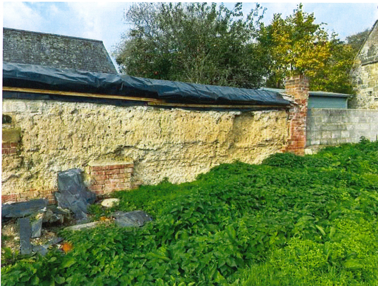
BOUNDARY WALL, THE BARFORD INN, BARFORD ST. MARTIN
