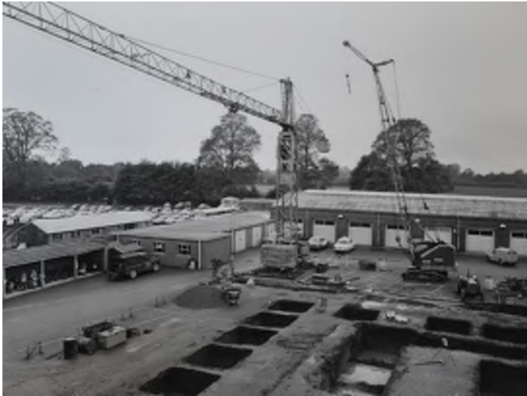
Photograph 8 – significant footings (right) for northern block to main building, dated 13 th May 1969 (Collection: F5/251/3)
