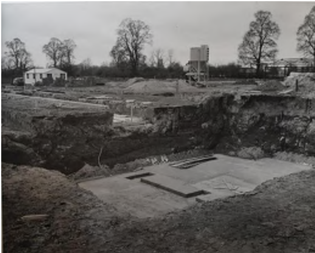
Photograph 7 - showing deep excavation for the footings of the buildings, dated 30th March 1961 (Collection: F5/251/3)
