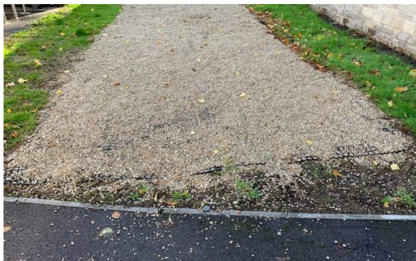
Photo 1 – Groundtrax Cellpave Access Track Example
