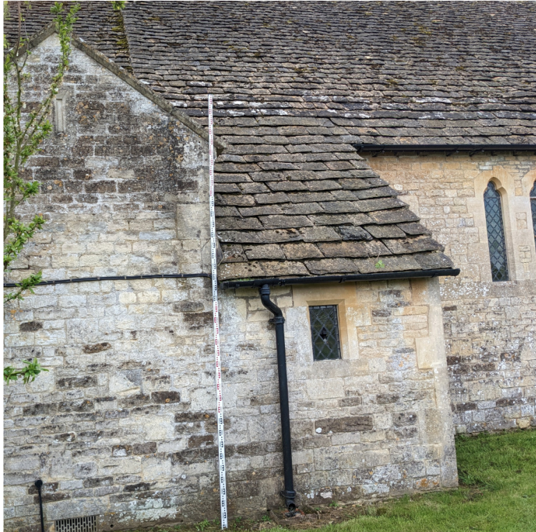
Image 7 – View of the Store (North side of Nave) - As Existing
