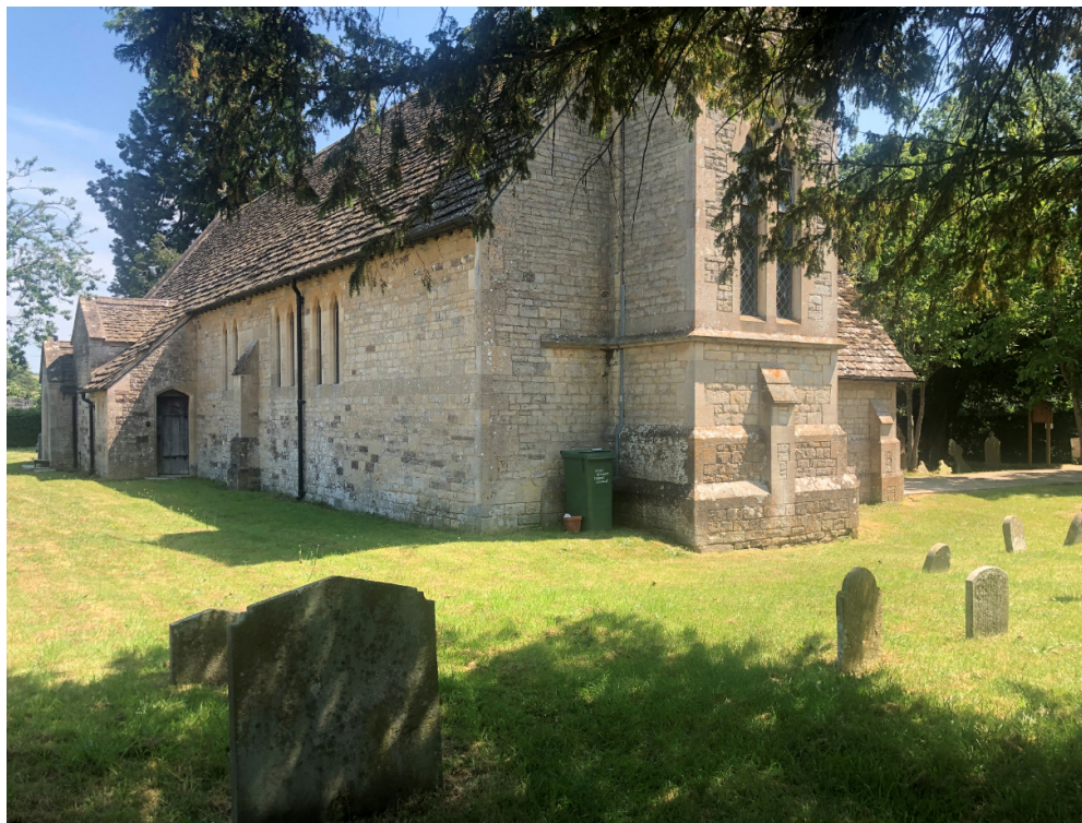
Image 4 – View of the Tower West Elevation & North side of the Nave – As Existing
