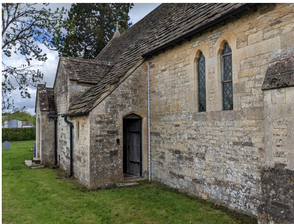
Image 6 – View of the Store (North side of Nave) - As Existing
