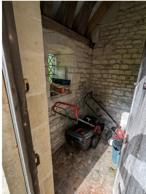
Image 8 – View inside of the Store (North side of Nave) - As Existing
