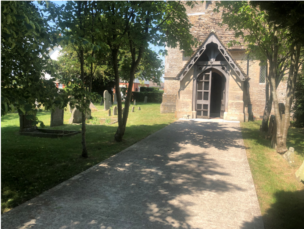
Image 3 – View of the South Porch and Path - As Existing
