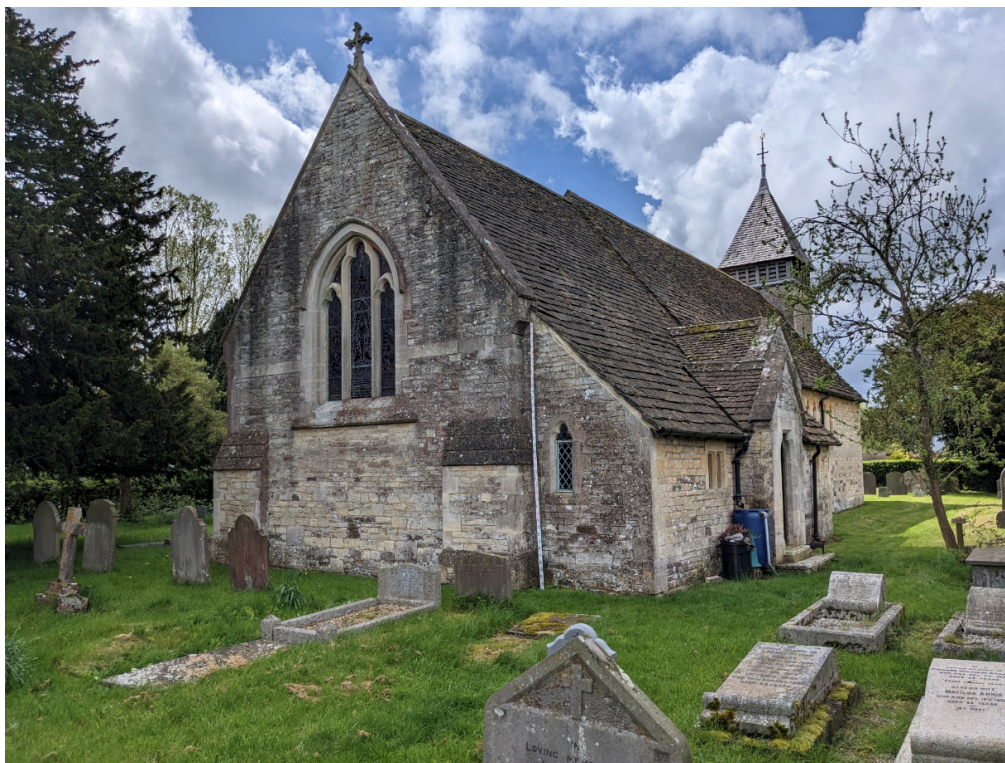
Image 5 – View of the East Elevation – As Existing
