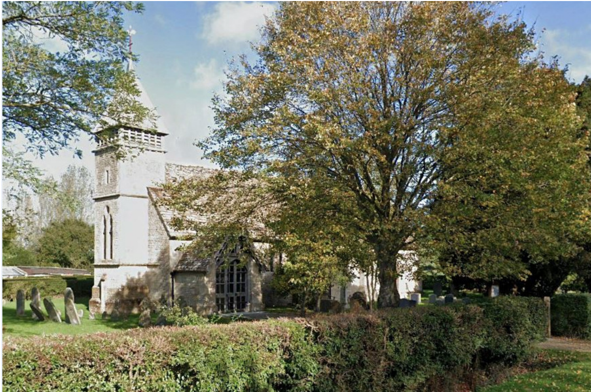
Image 1 – View of the South Elevation from the main road – As Existing
