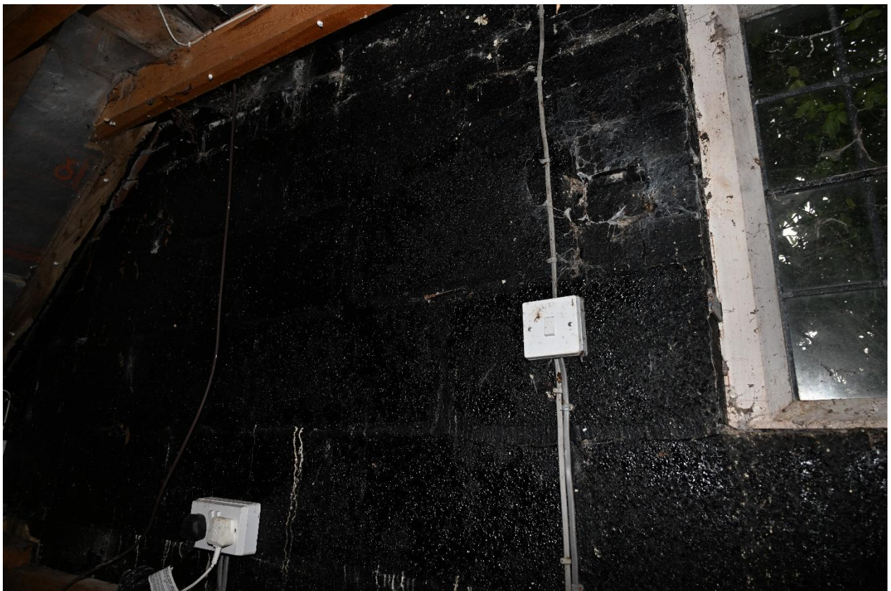
Image 4 Damp and water ingress
