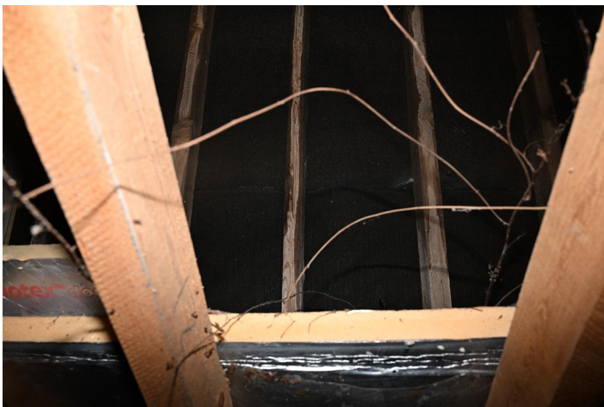
Image 2 Roof Structure Image 1 – Plant ingress
