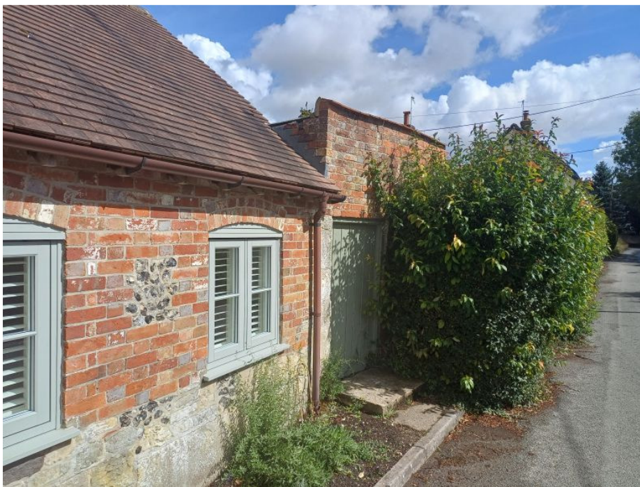
Wall – rebuilt following approval 2016 with gate. Neighbours outbuilding in foreground
