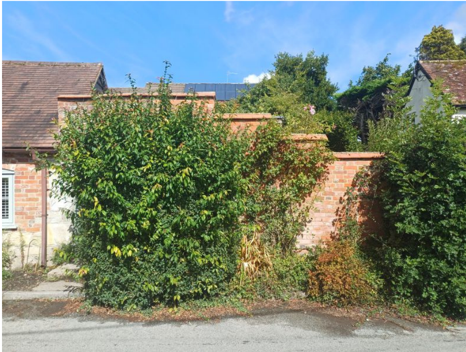
Wall – rebuilt following approval 2016
