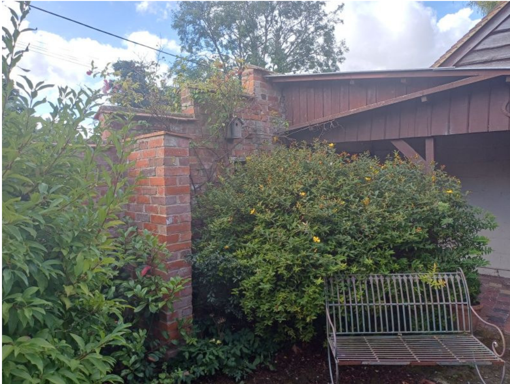
Wall with buttress in foreground added following 2016 planning approval. Lean to structure built between walls and neighbours outbuilding behind
