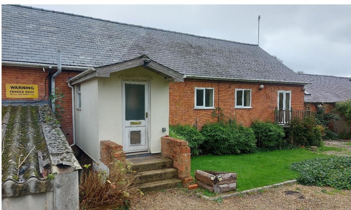
Figure 8: Showing part rear (SW) elevation with existing main flat entrance through porch
