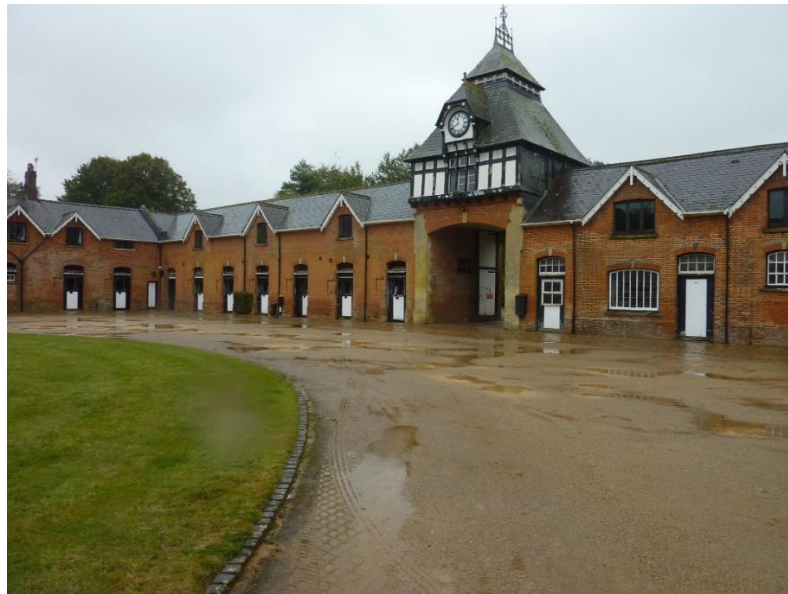
Figure 2: Photograph showing main entrance to listed stables (taken within quadrant)
