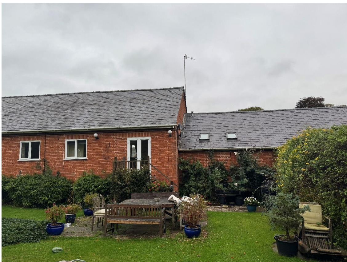
Figure 9: Showing existing part SW elevation – flat extends beyond the dividing boundary treatment on the right of this photograph
