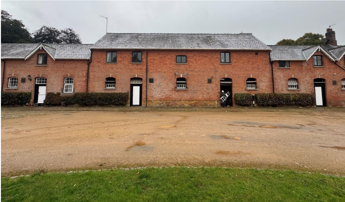
Figure 6: Showing existing NE elevation of the southwestern wing.
