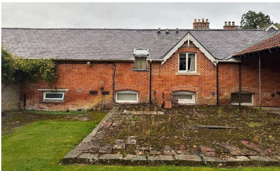
Figure 7: Showing part of the rear elevation of the Library Flat towards the left, (gabled dormer is beyond the flat's extent)
