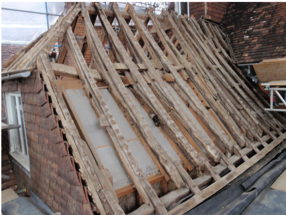
Fig 1 View of east side of roof over Bedroom 3.
