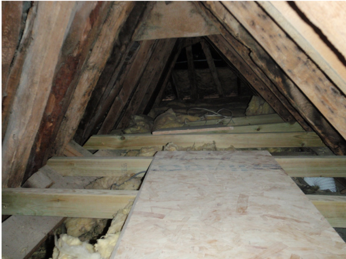
Fig 1 View from the roof access into the loft space over Bedroom 3.
