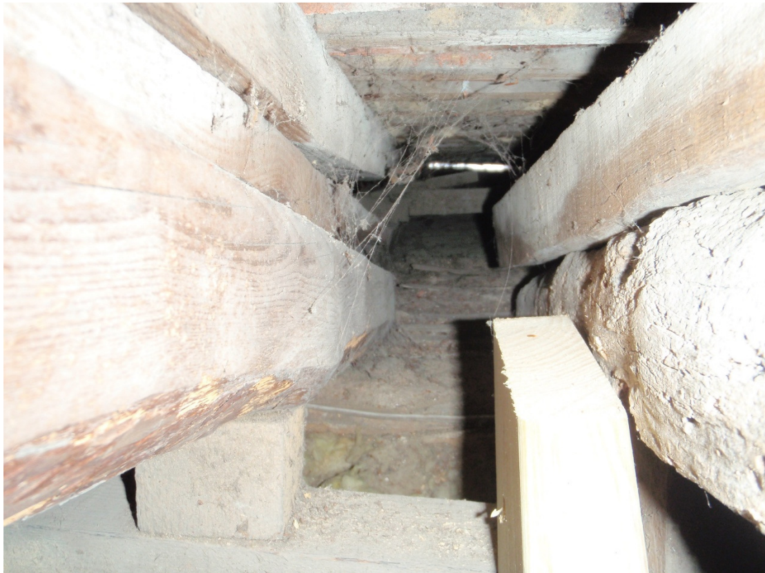
Fig 5 Packing of rafters on east slope looking down the skilling.
