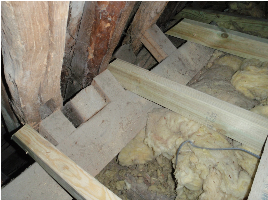
Fig 4 Packing out between rafters and more modern purlin on east side of roof. Note horizontal members added only for temporary access.
