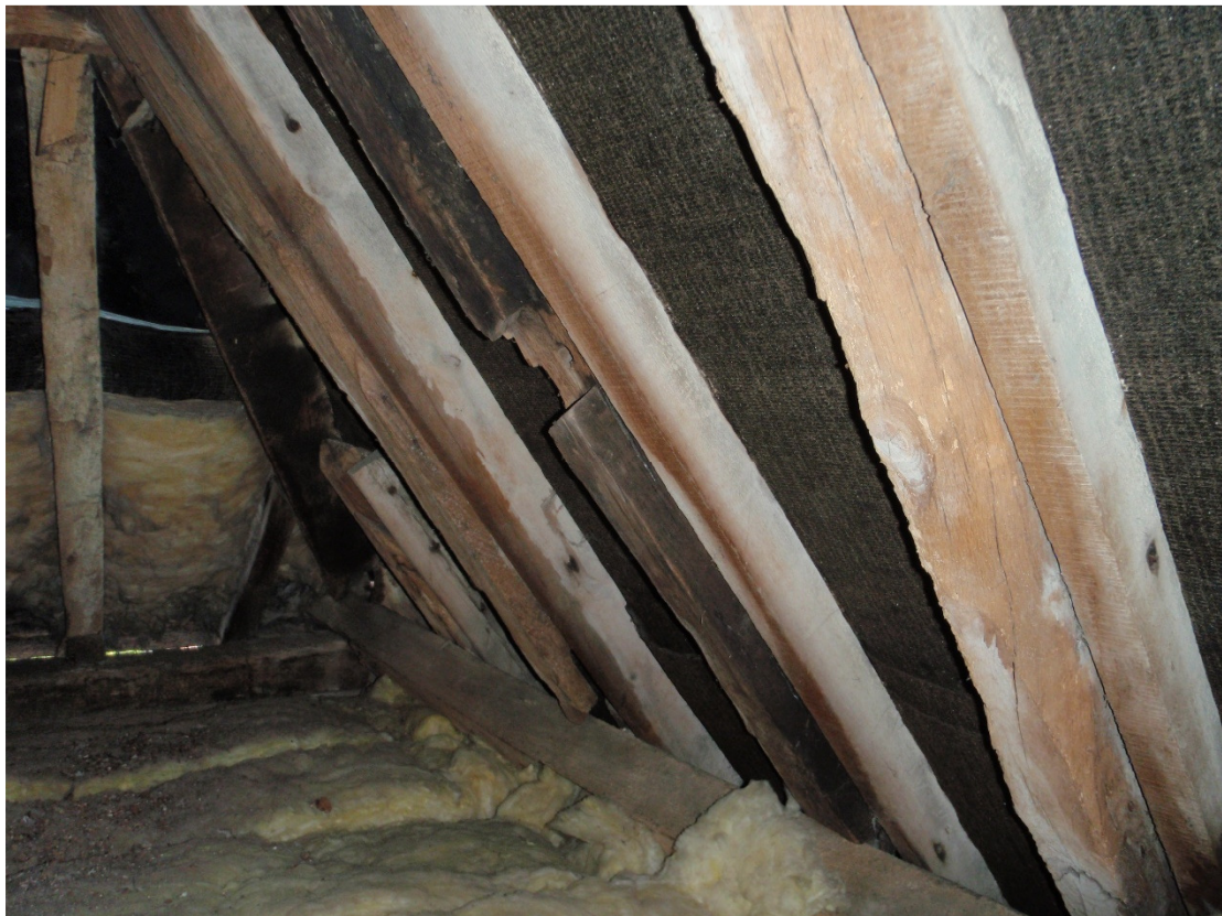
Fig 2 Additional rafters against the original ones on the west roof slope.
