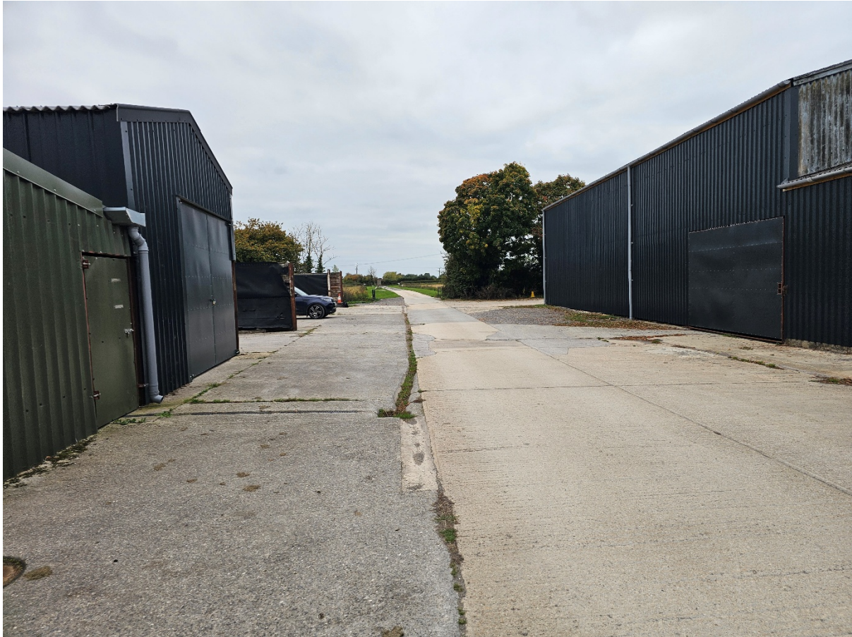
Looking South West towards Devizes Road entrance to Lower Farm / Rowdey Cow
