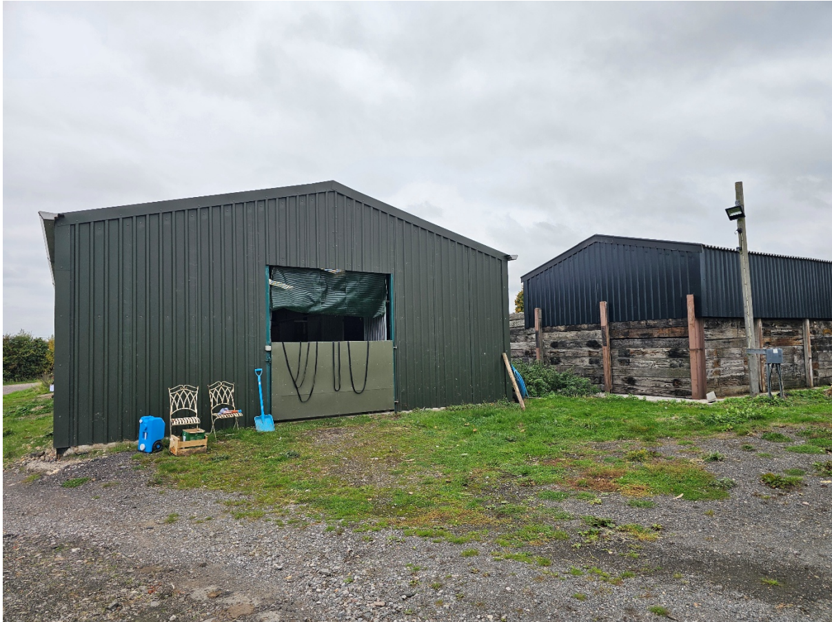
Existing buildings South East / East (behind) the proposed Padel Court facility
