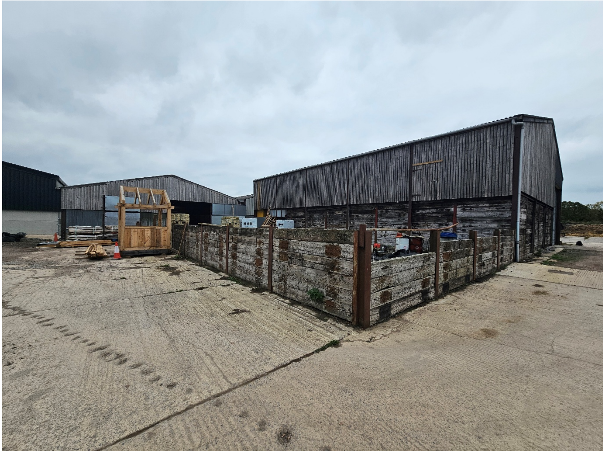
Existing buildings North West (opposite) the proposed Padel Court facility
