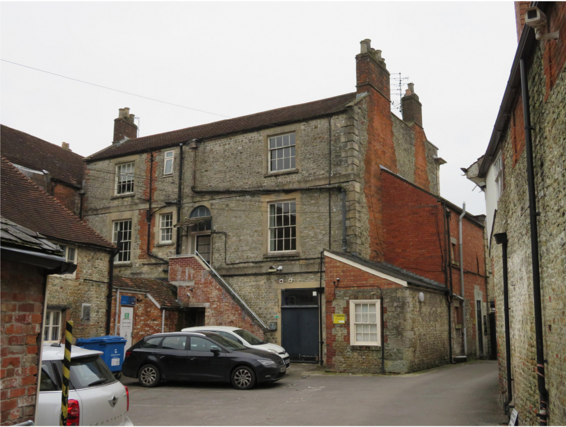
PHOTO OF EXISTING BUILDING REAR
