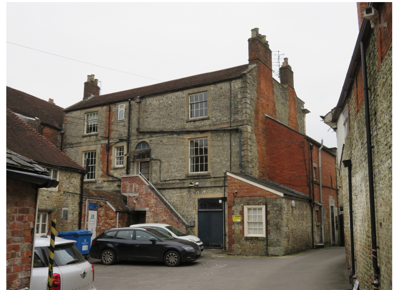
FIG.6 Looking at rear of building
