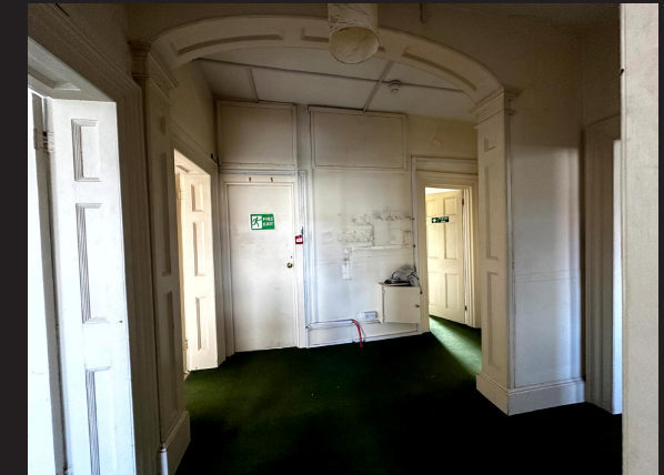
FIG.9 Central Lobby area
