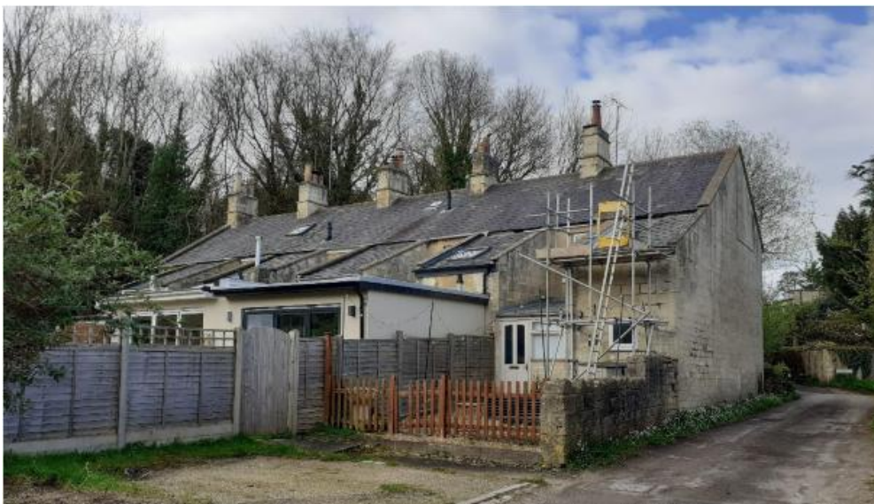
Figure 2 Rear of The Tynings showing differing extensions and skylights
