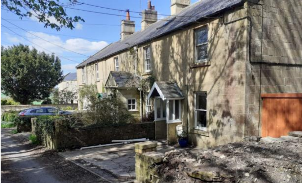
Figure 1 Front of The Tynings showing various modifications including additions of porches
