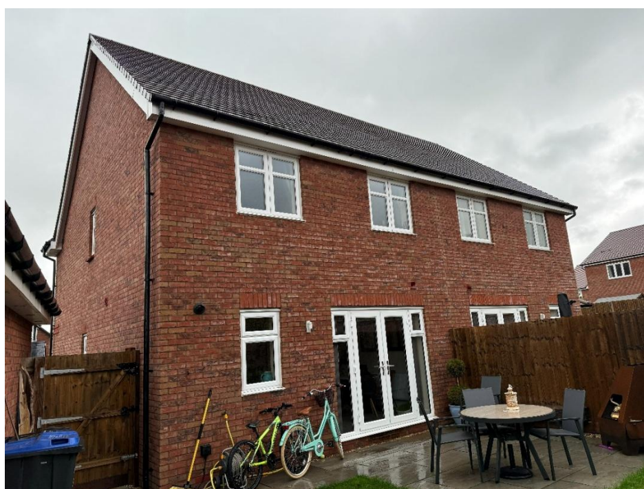
Figure 4 - Rear Elevation of no. 8
