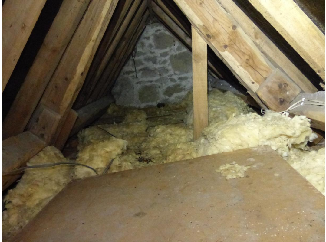
Figure 15 – Northern section of loft void viewed from access hatch
