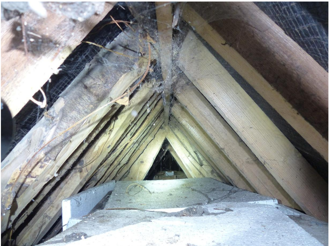
Figure 16 – East-west running loft void viewed from access
