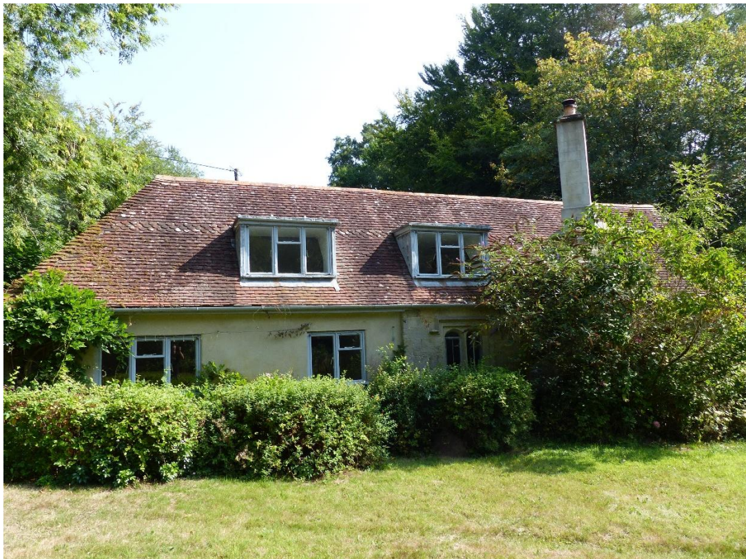
Figure 5 – Southern aspect of Wincombe Lodge
