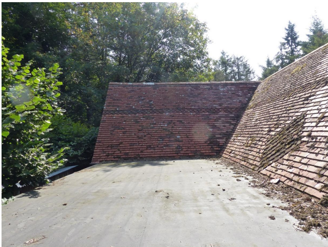
Figure 8 – Area of flat roof forming the northwest part of the property
