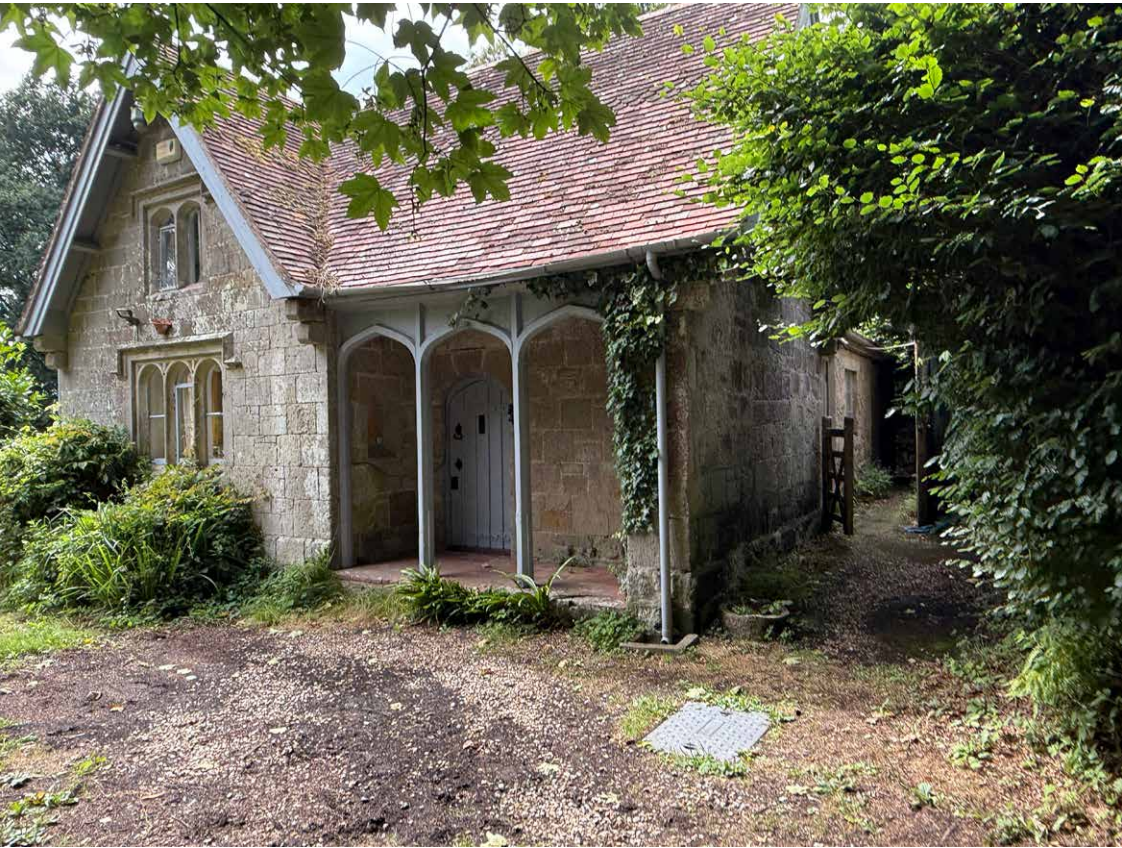
Pictures showing the existing building on site
