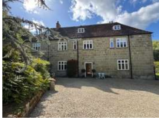
Fig 2 – View of site looking from the North.
