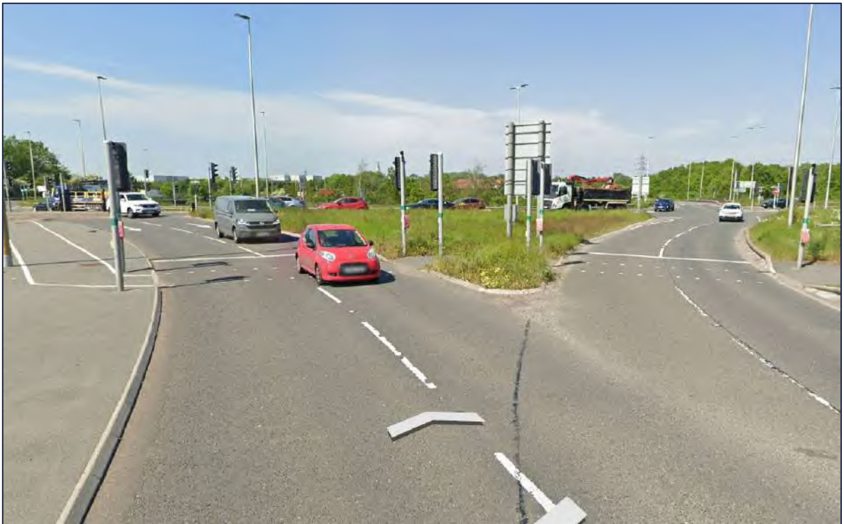
Figure 5.1 – Existing Pedestrian Crossing at Junction 16
