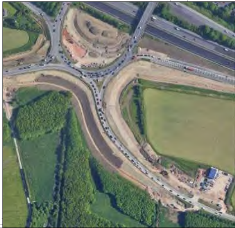
NORTH SOUTH AERIAL VIEW
