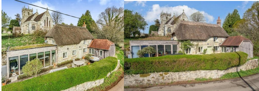
Picture of the cottage before the increase in chimney height in 2022 (left) and after being raised by 8 brick courses in 2024 (right)
