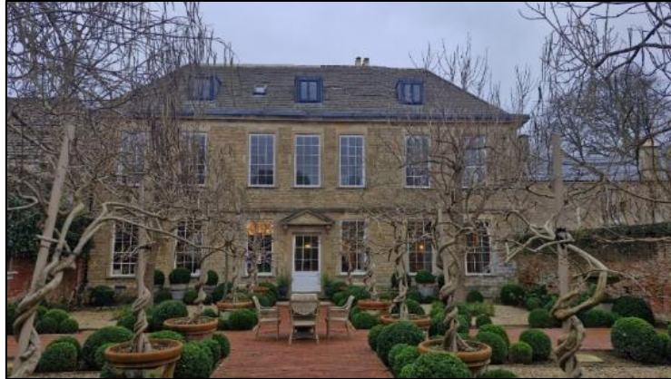
Plate 14. Rear (west) elevation of Shaw House
