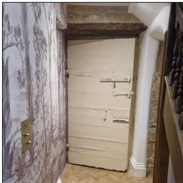
Plate 24. Original External Service Door
