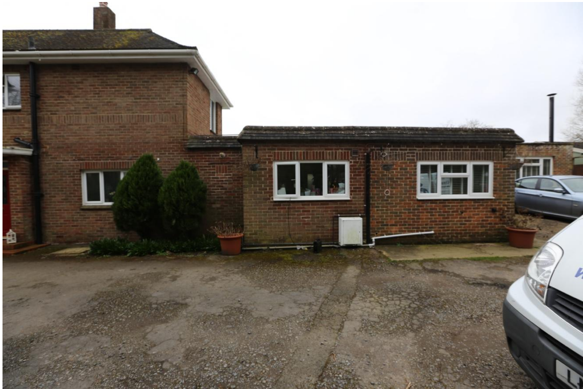
Lydiard Farm - View looking at the front of the property, right side.
