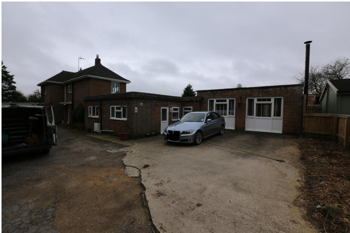
Lydiard Farm - View looking at the front of the property, right side and annex
