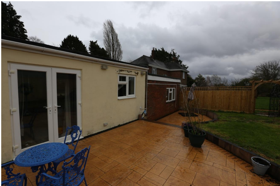
Lydiard Farm - View looking the rear of the annex, with main house in background
