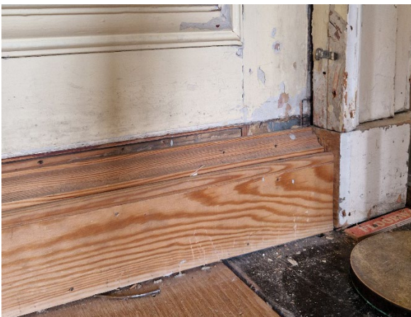
South wall below PS-3.2
