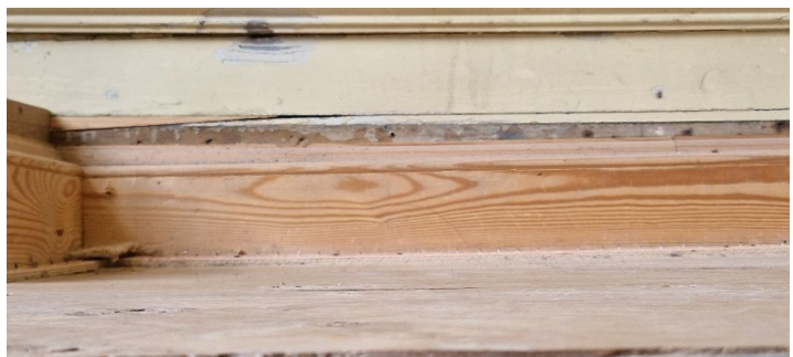
East wall below PE-2.2
