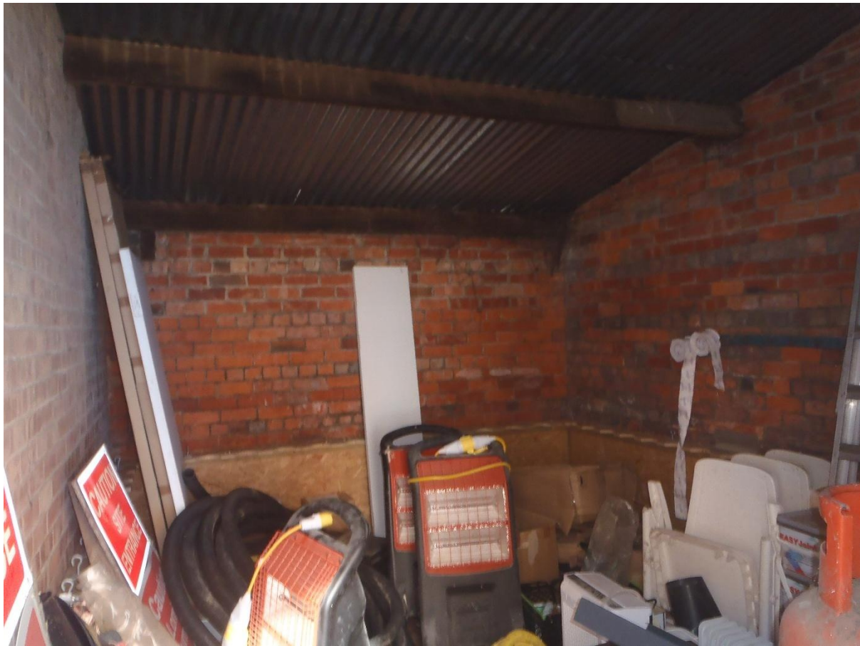
Photograph 8: showing a view inside of the storage sheds
