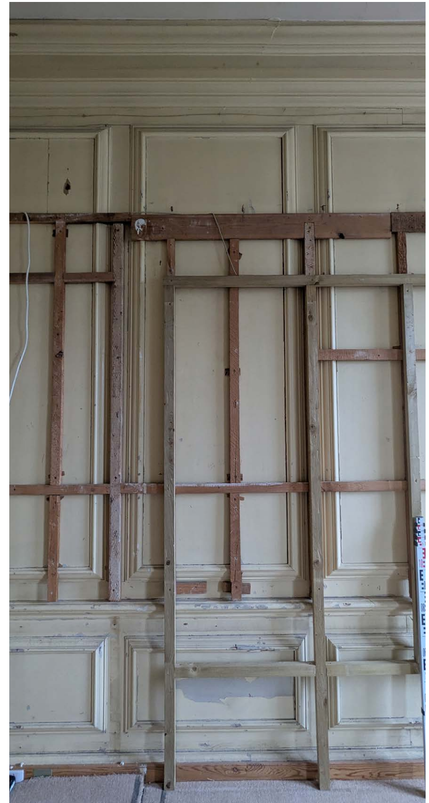
Bolection-moulded upper and lower panels separated by dado rail
