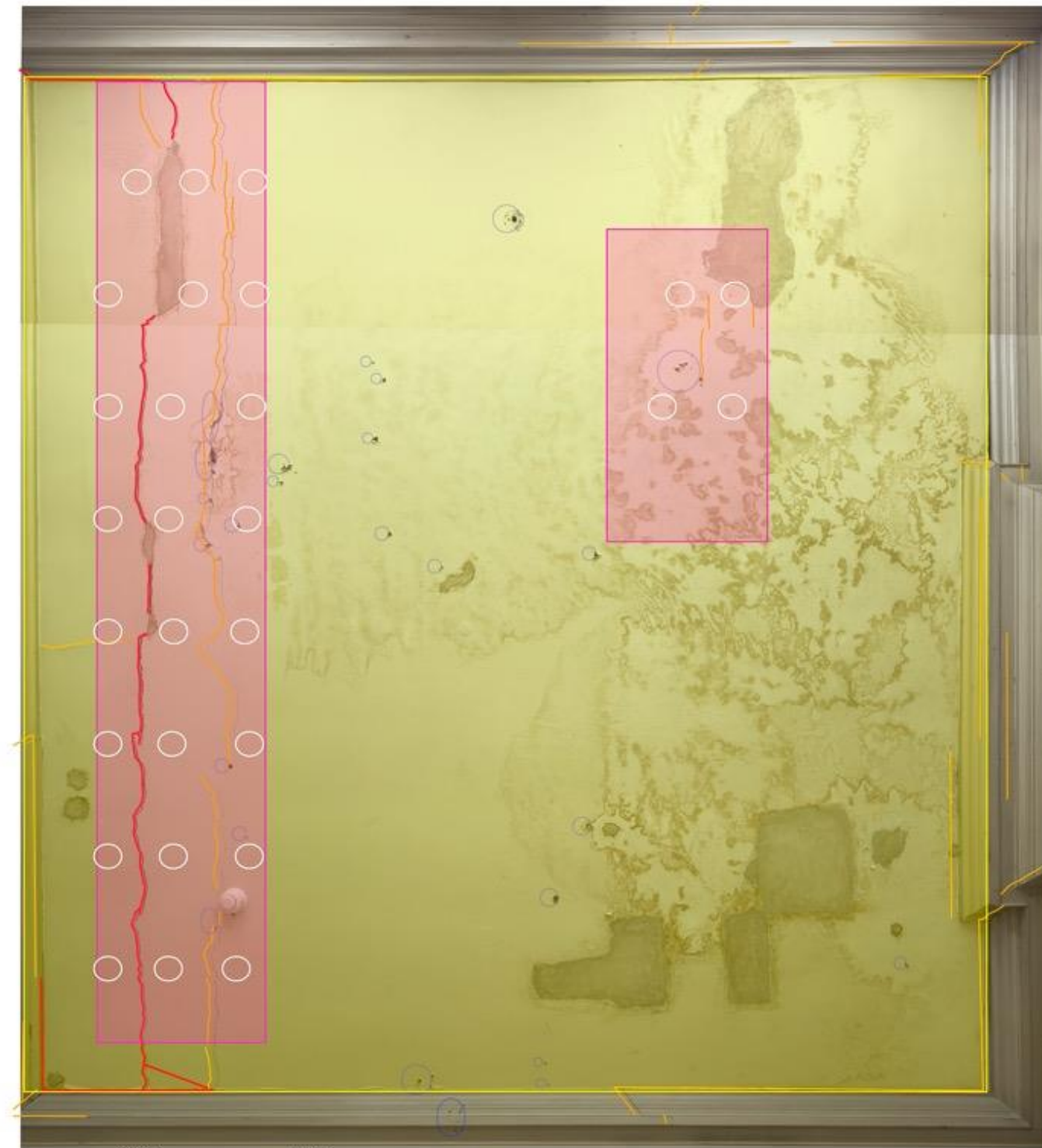
Reflected ceiling plan from Cliveden Conservation report. Areas in red to receive recessed washer support
