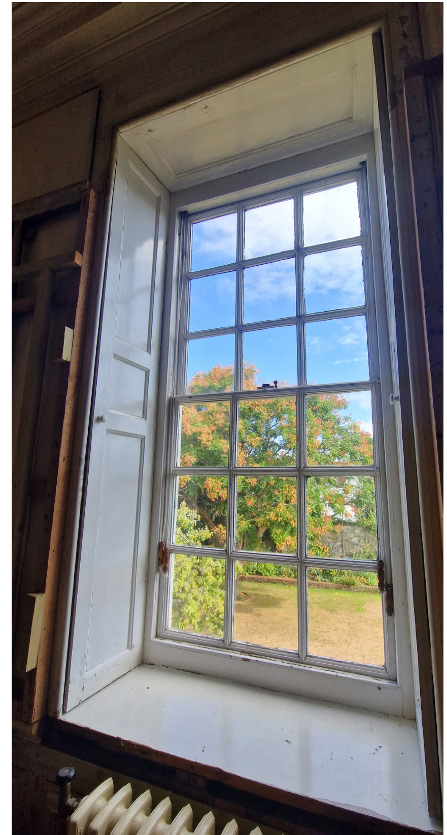
Window with shutters open
