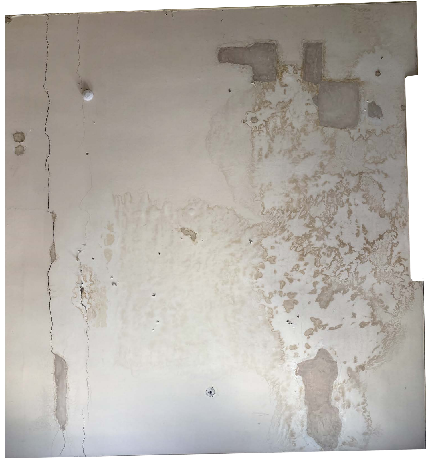
Existing condition of ceiling
