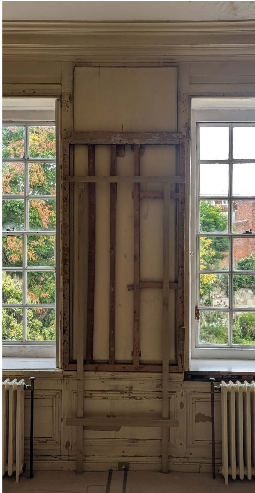
'Mirror panel' between windows
