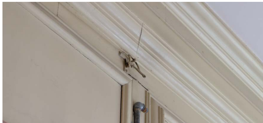
Remnant of mechanical bell pull system
