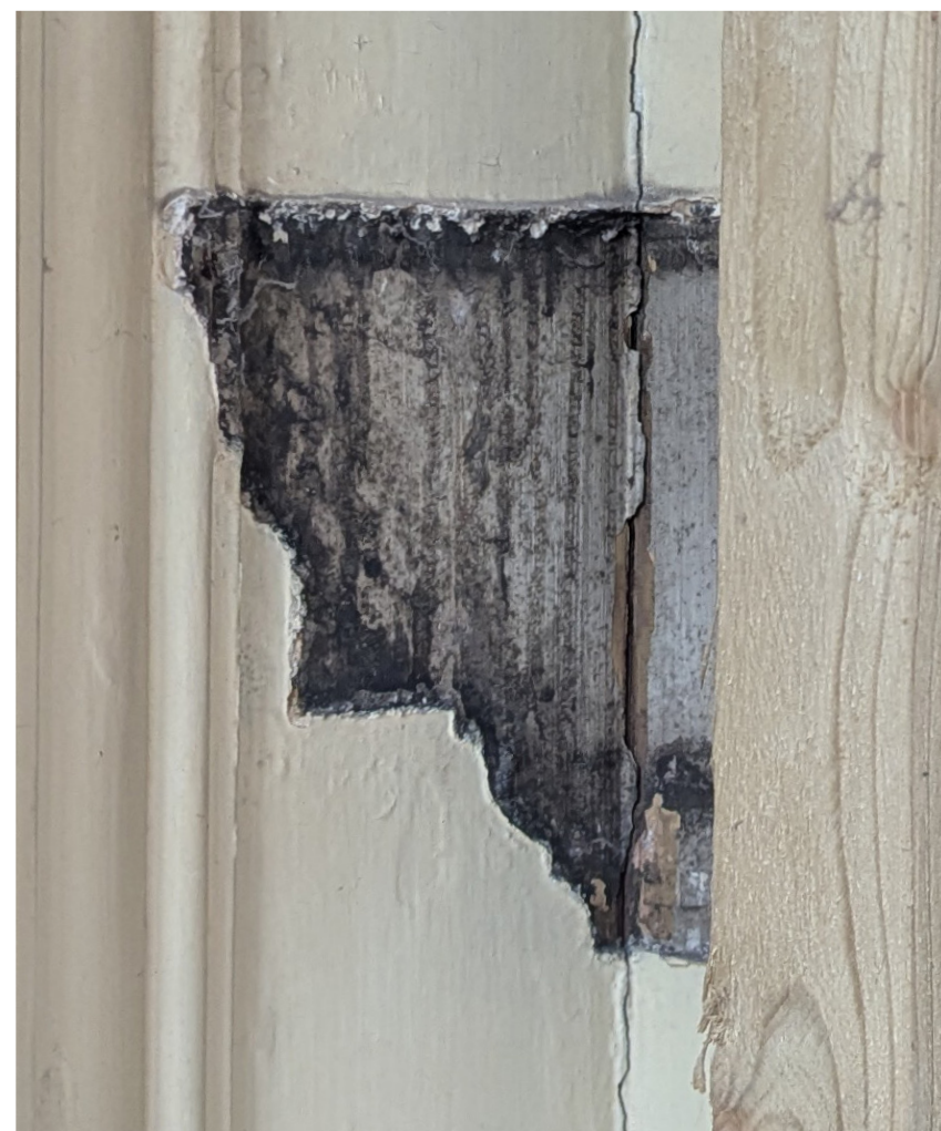
'Ghost profile' of mantle shelf at left hand side of fireplace
