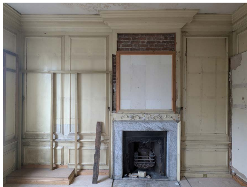
Existing condition: East wall
