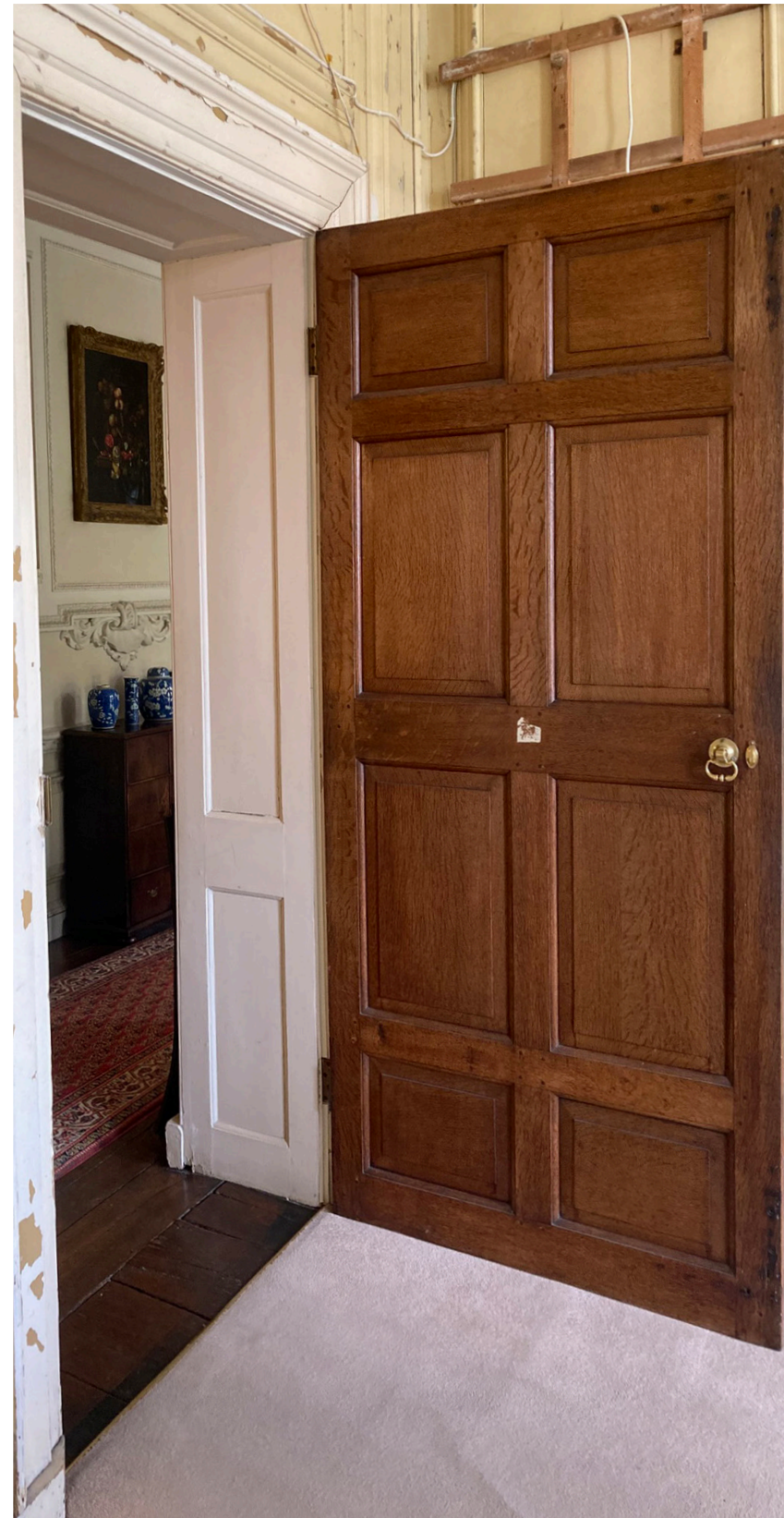
Door, looking into hallway
