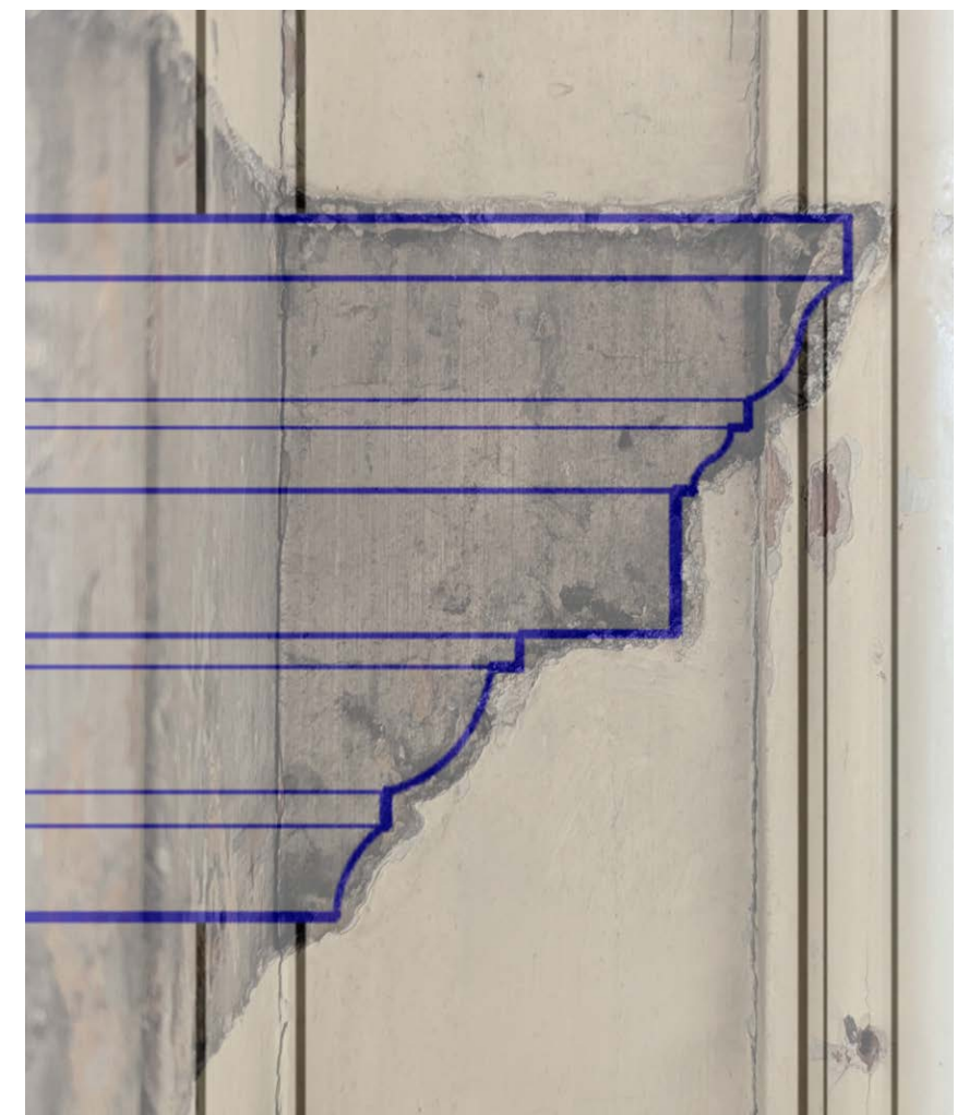
Proposed profile of reinsrated mantle shelf superimposed on 'Ghost profile' at right hand side of fireplace
