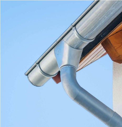
Rainwater goods - metal
