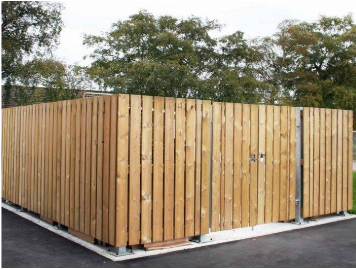
Commercial bin store for no. 53
