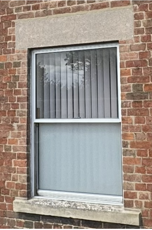
EX aluminium framed sash window
