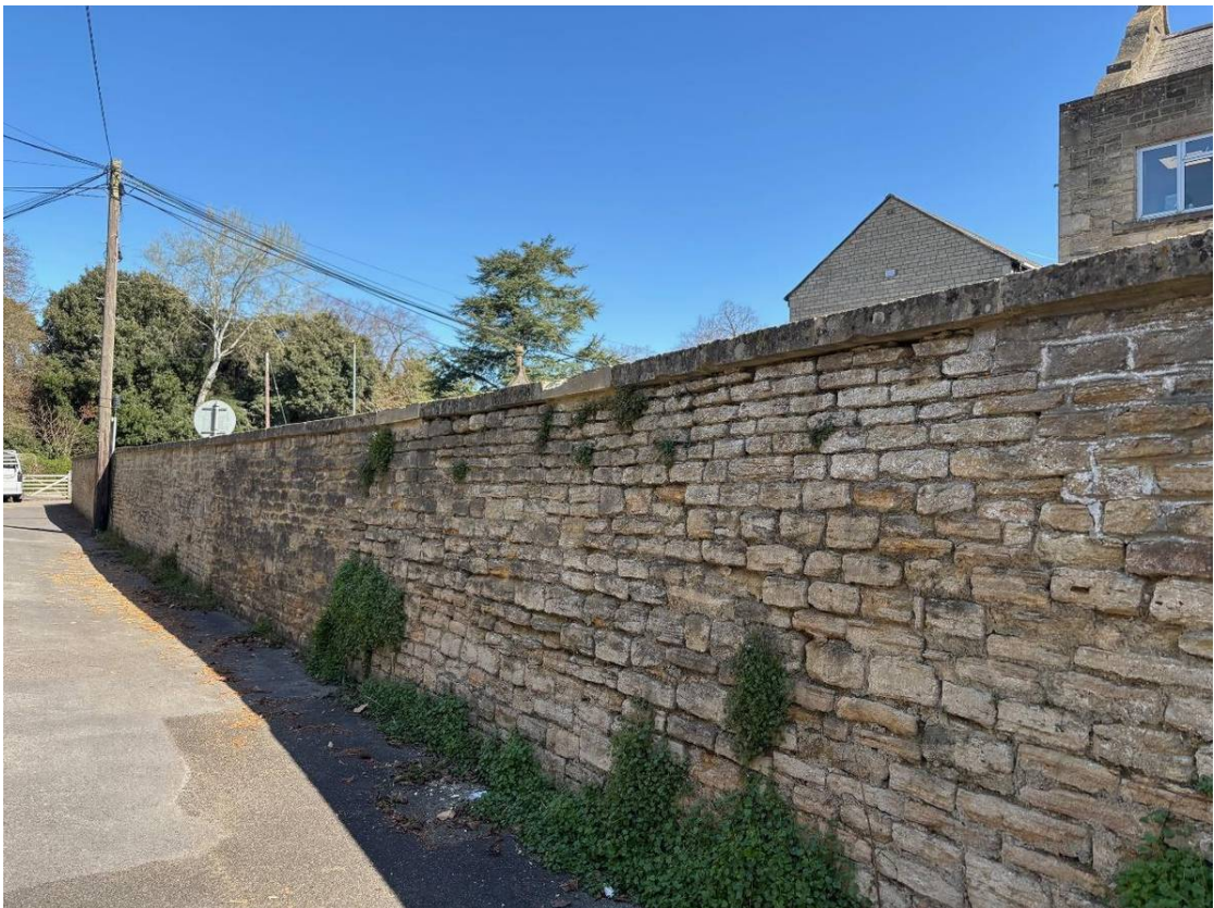
Fig.13 Coursed rubble stone wall bounding the east side of the long driveway (separation from the hospital site)
