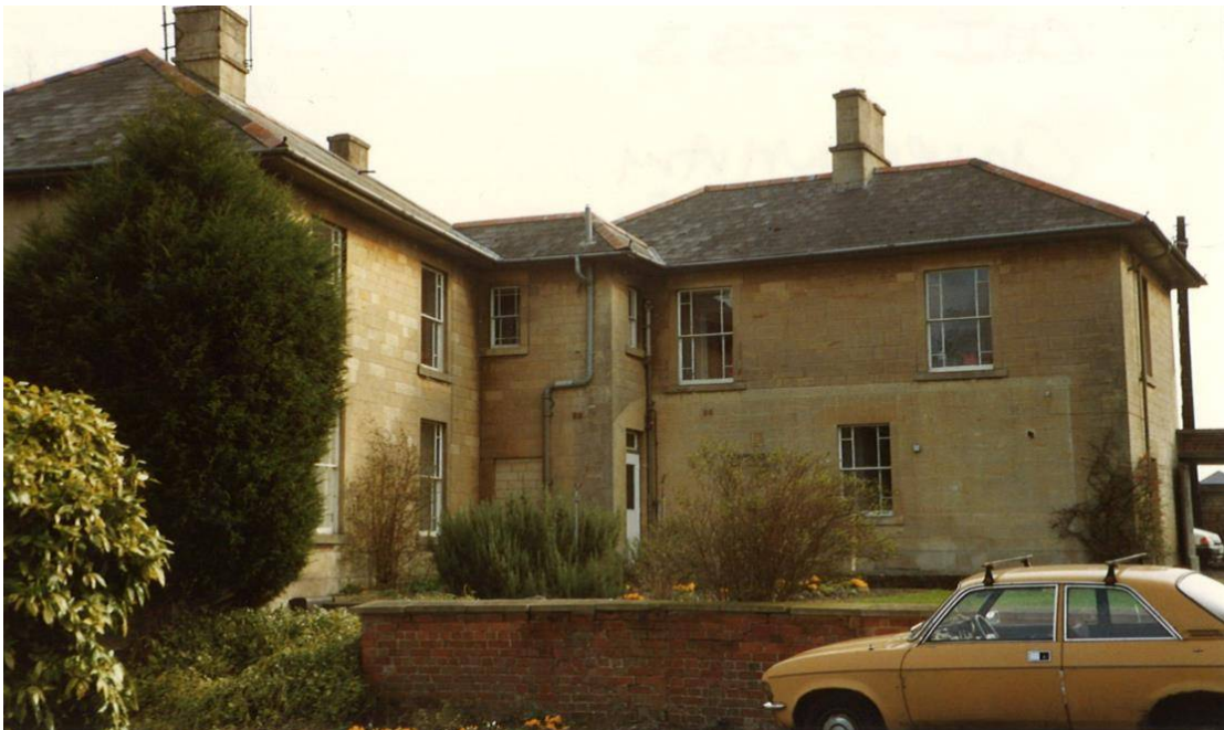
Fig.30 Photograph from 1980, prior to the external staircase (Wiltshire Buildings Record)
