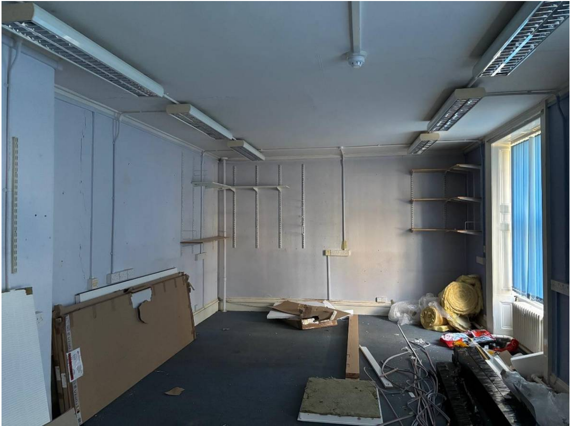
Fig.16 Principal ground floor room of No.51 – modern ceiling, light fittings and ducting
