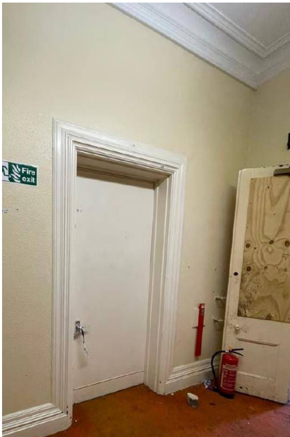
Fig.8 Example of an over-boarded panelled door and original architrave within No.53
