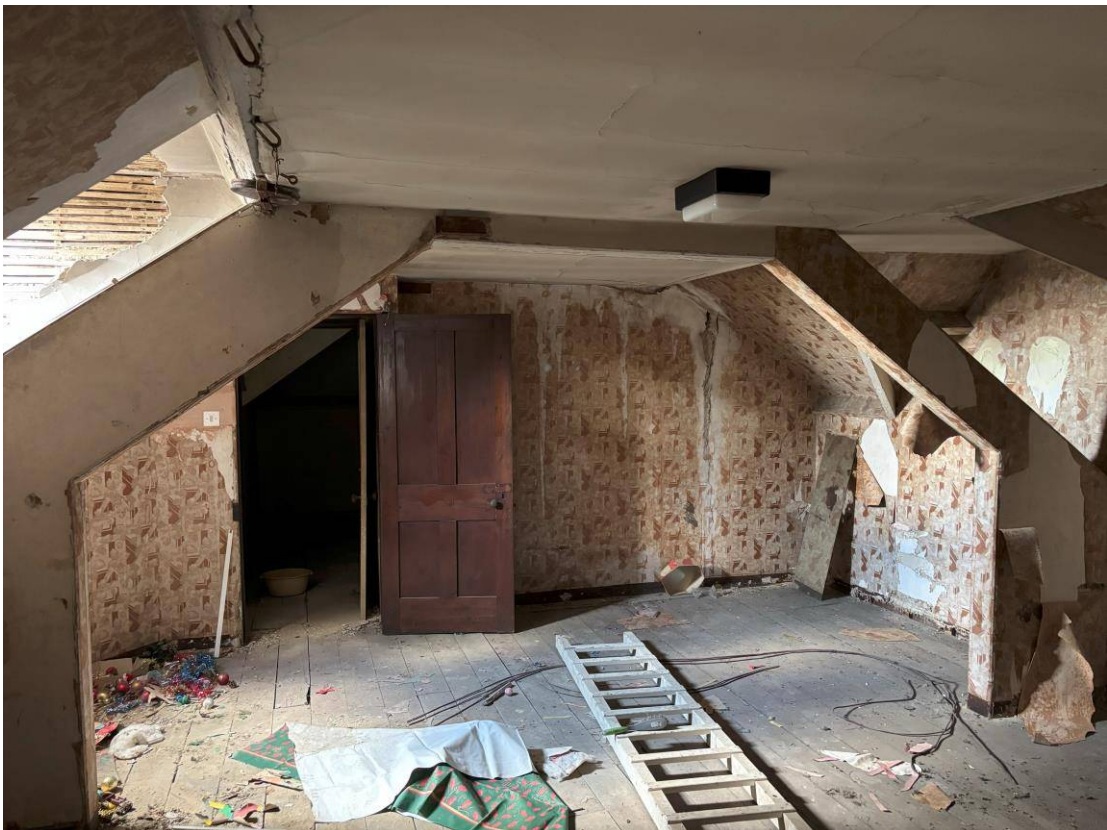
Fig.10 One of the attic rooms within No.53 – original floorboards and lath and plaster ceilings
