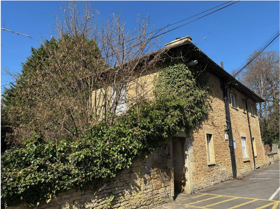
Fig.12 East side of No.51 as seen from the long, eastern driveway
