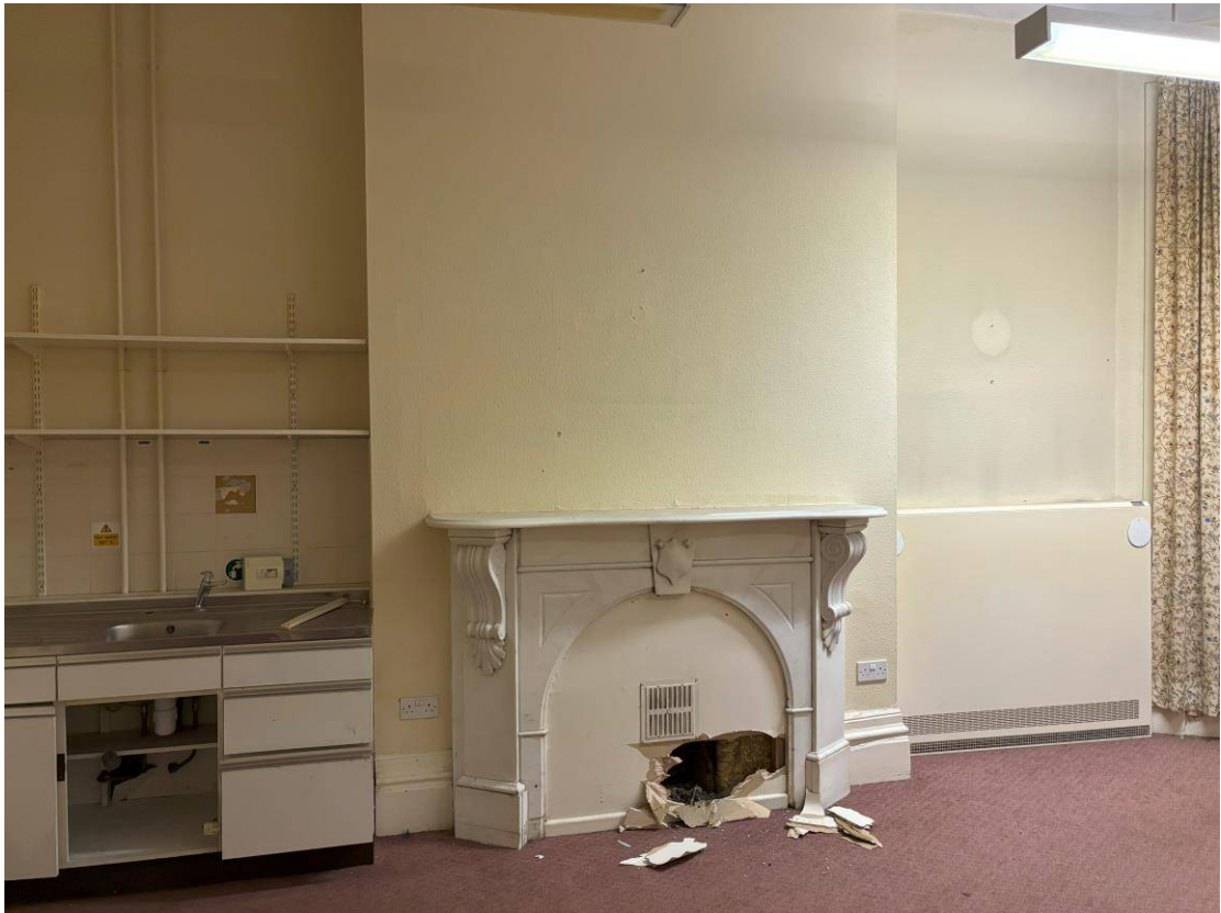
Fig.7 Original fireplace in the main ground floor room of No.53
