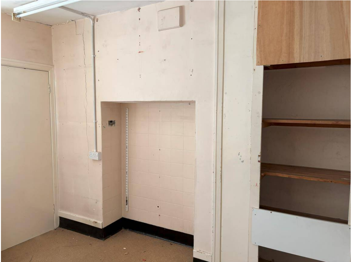
Fig.17 Example of one of the plainly decorated rooms within the service range of No.51
