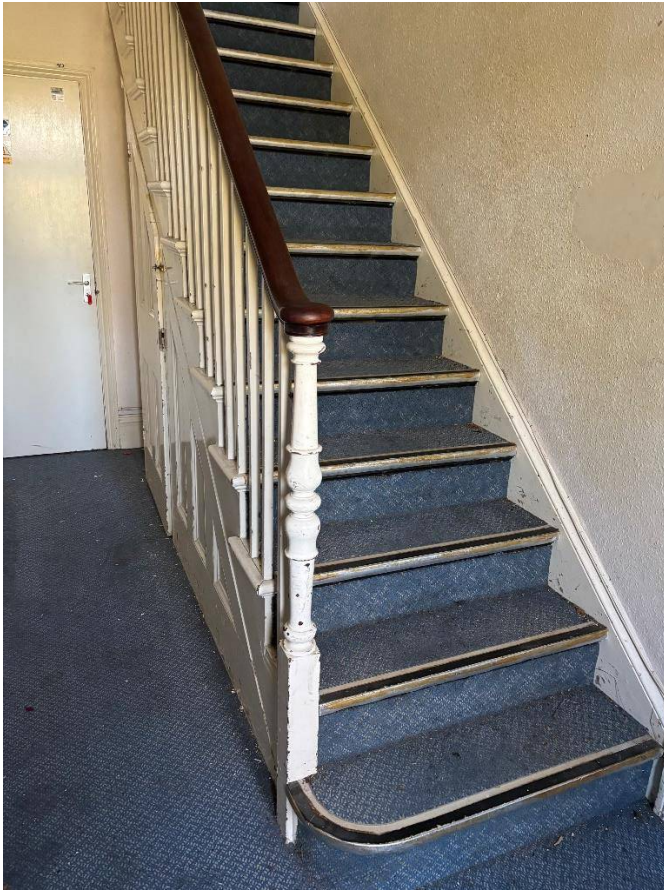
Fig.14 Staircase in No.51
