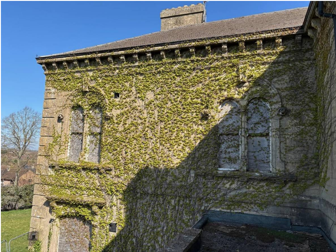
Fig.4 View from the roof of the modern link towards the ivy-clad south wall of No.53
