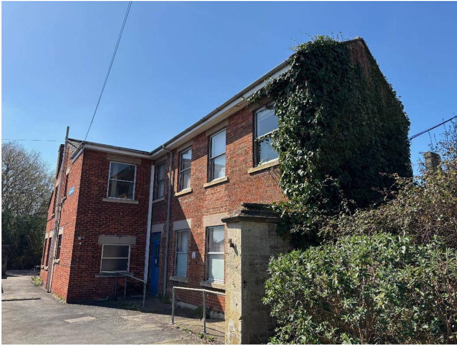
Fig.18 East side of No.49
