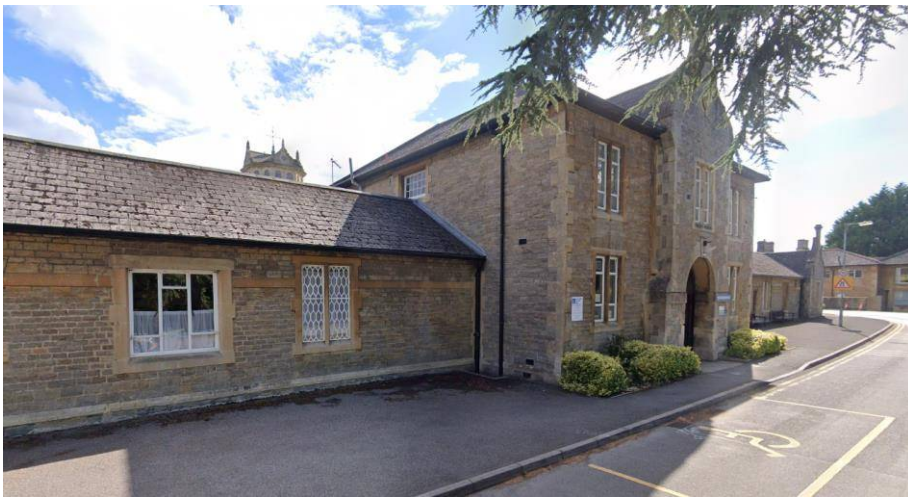
Fig.20 Front of the Chippenham Community Hospital
