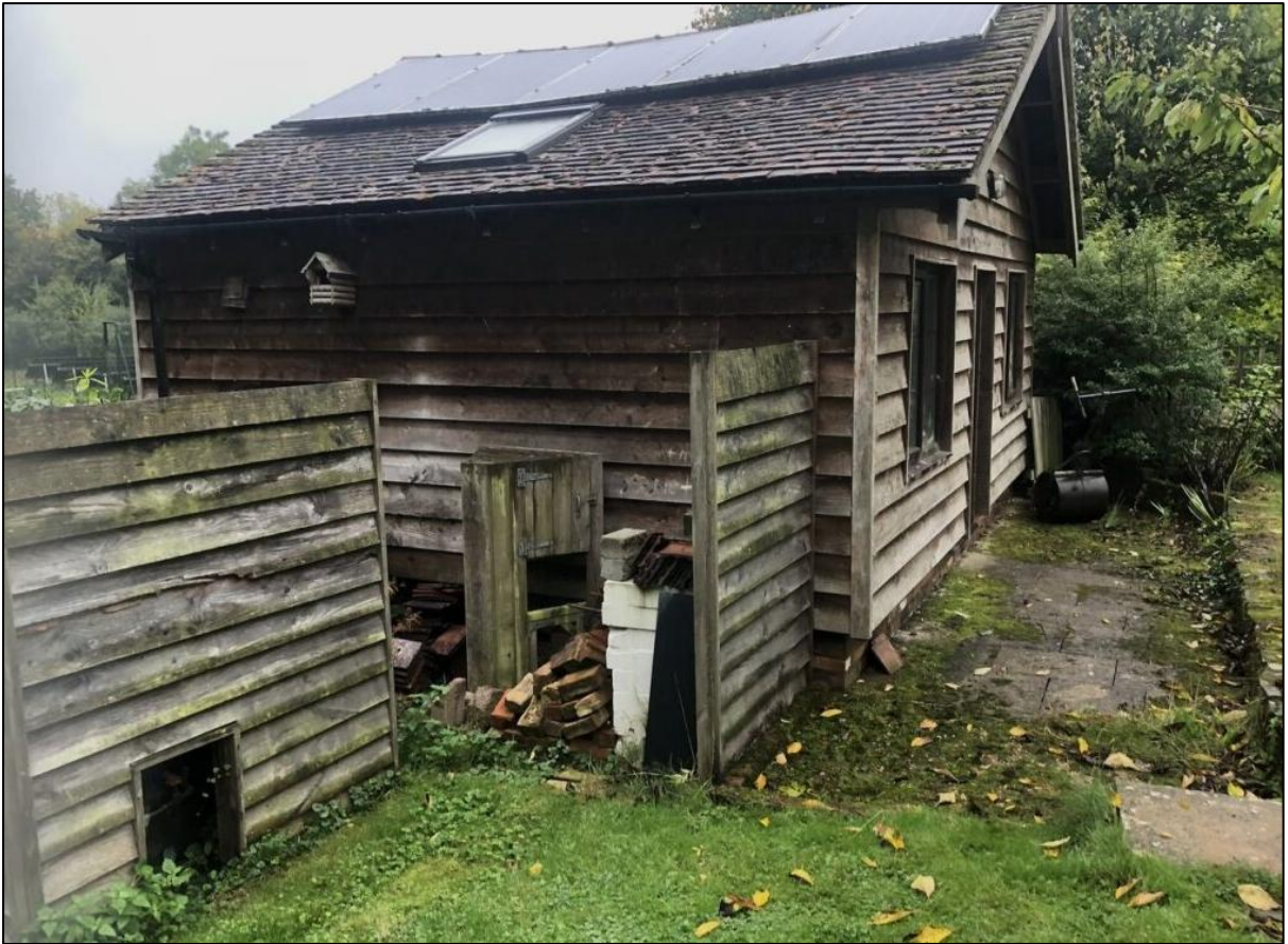
Photographs of ancillary outbuilding to be demolished
