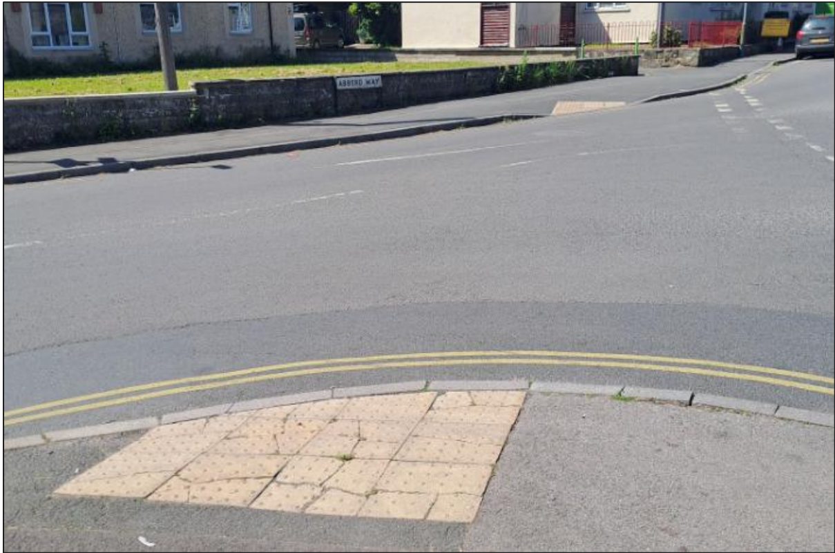
Image 24 - Crossing Facilities at Abberd Way/Oxford Road Junction
