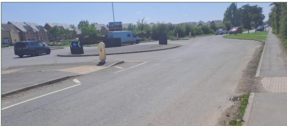
Image 35 - Pedestrian Crossing Facilities at Oxford Road/Sycamore Drive Roundabout
