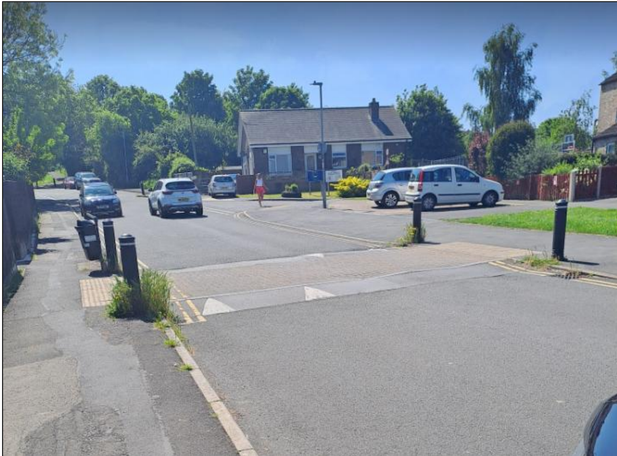
Image 21 - Pedestrian Crossing Facility on Prince Charles Drive
