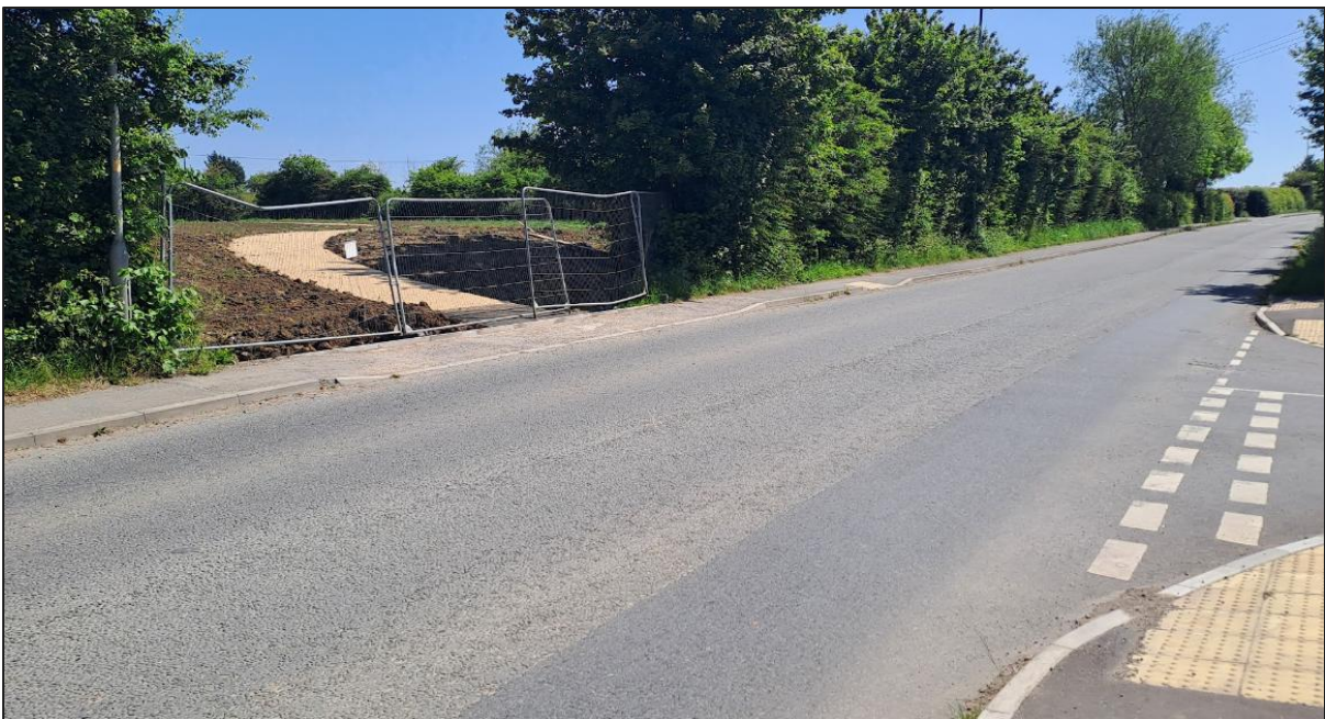
Image 11 - Footway Connection to Sand Pit Road
