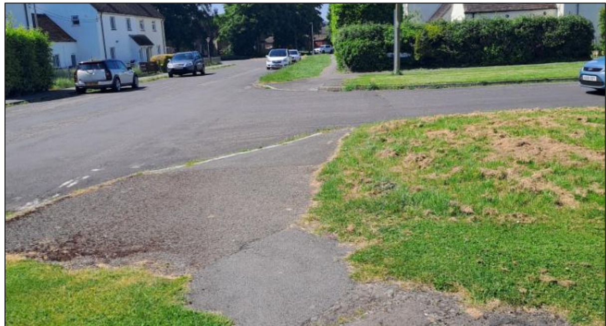
Image 18 - Crossing Point at Abberd Way/Woodhill Avenue
