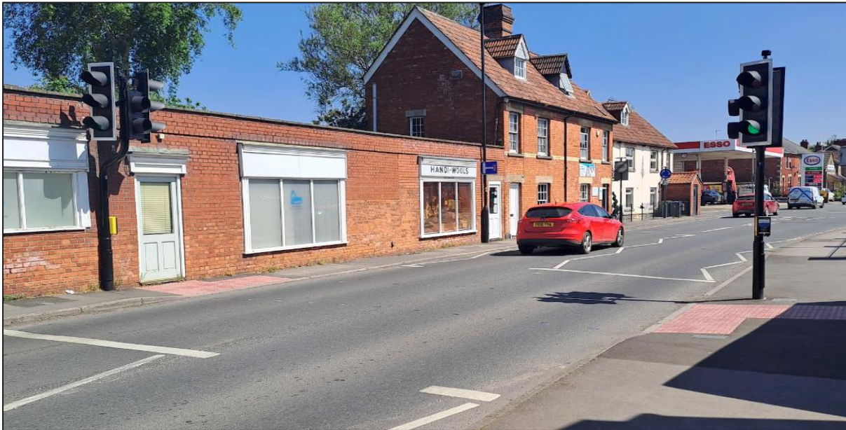
Image 26 - Signalised Crossing of Oxford Road
