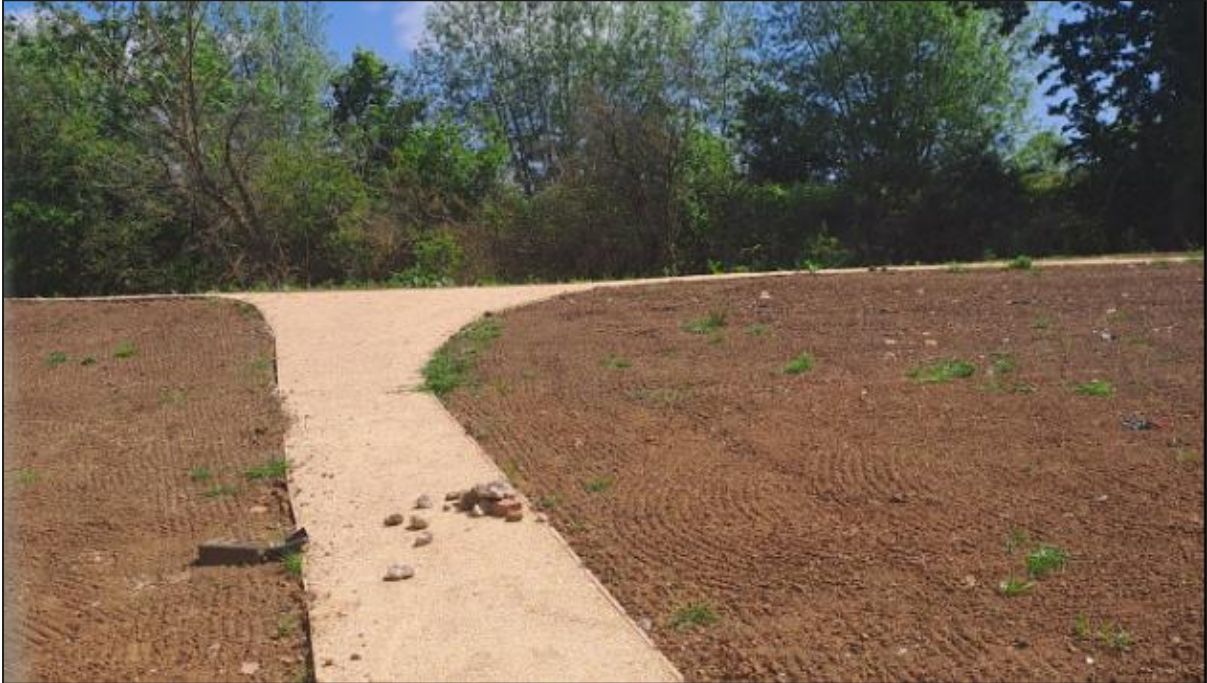
Image 10 - Segregated Footways in Neighbouring Development
