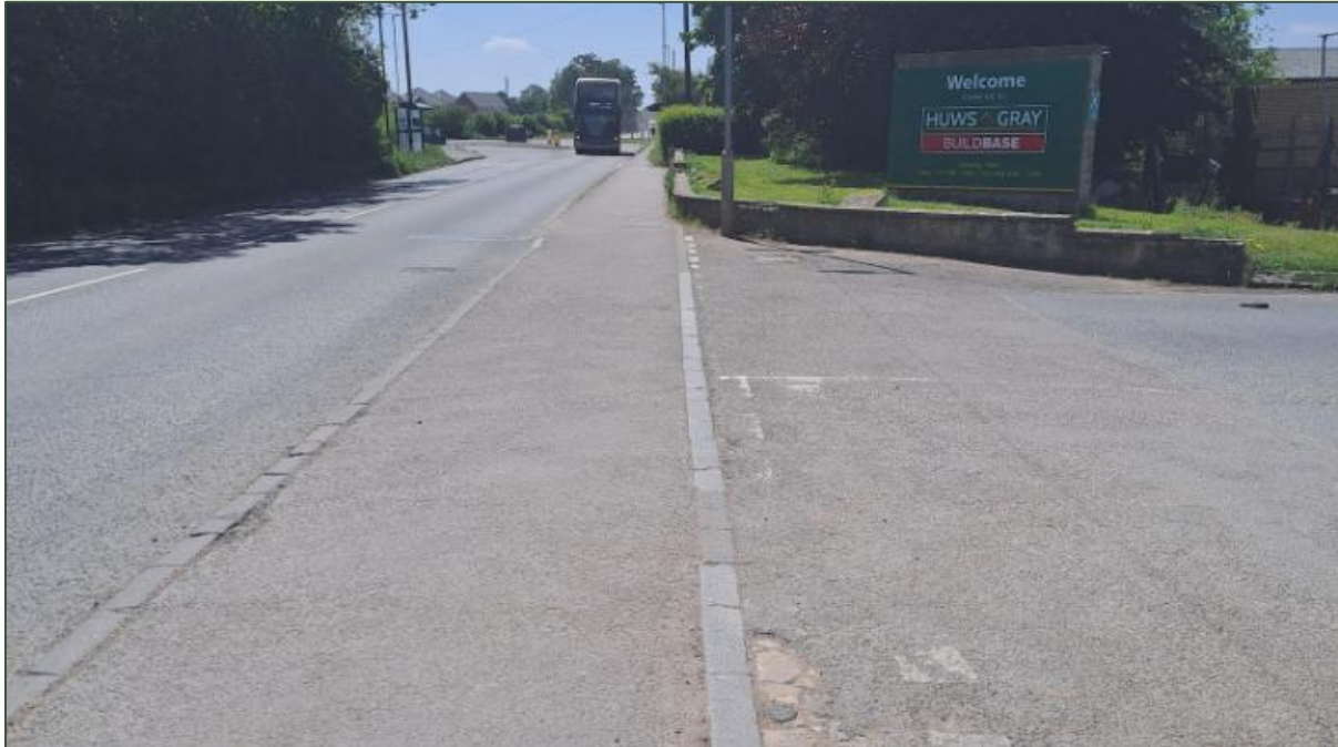
Image 36 - Huws Gray Buildbase Crossover Arrangement
