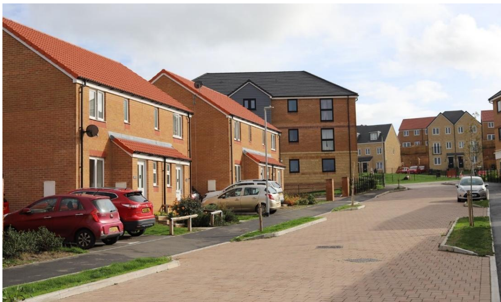
Figure 4.9: Typical residential properties within LLCA2
