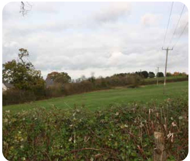
Fig. 21: Existing overhead electric transmission lines running north-south through the western field.
