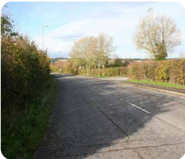
Fig. 13: Existing access junction on Sand Pit Road , looking west.
