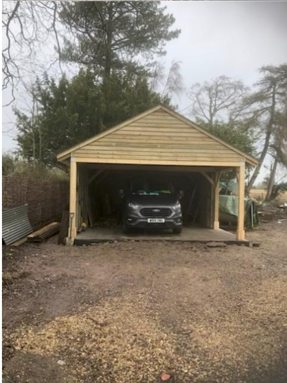
As built originally.
