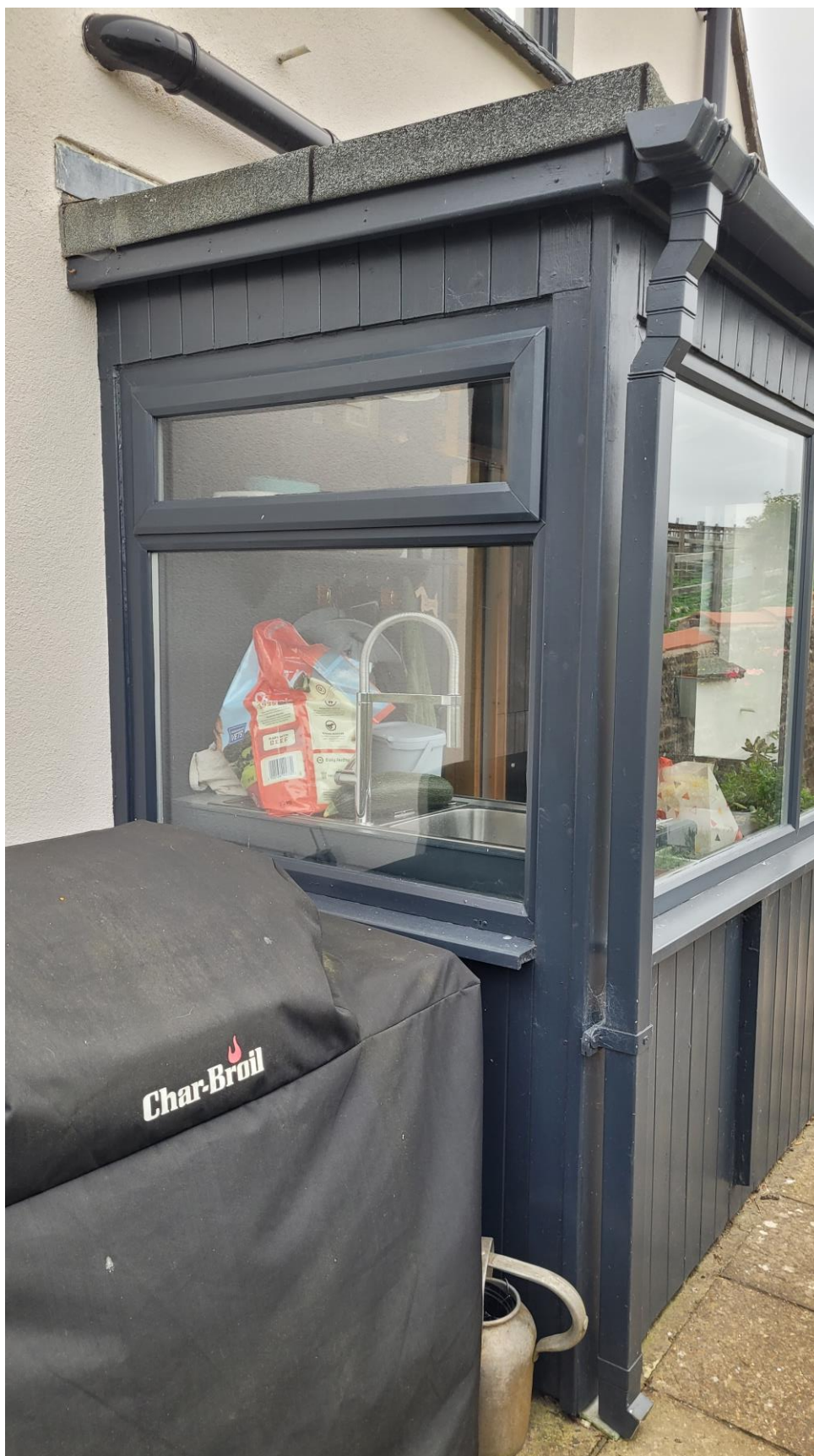
Fig. 4 – East elevation of existing utility room
