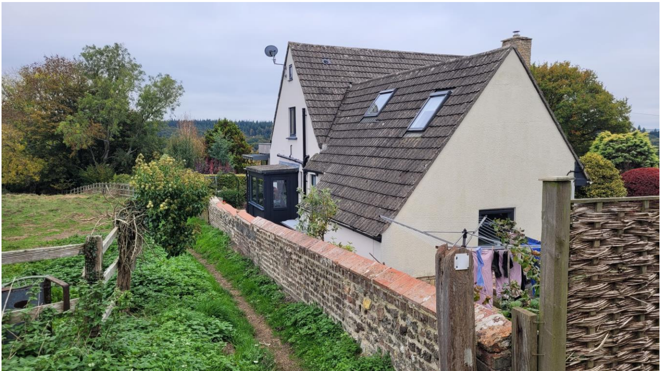
Fig. 2 – Rear of property viewed from West
