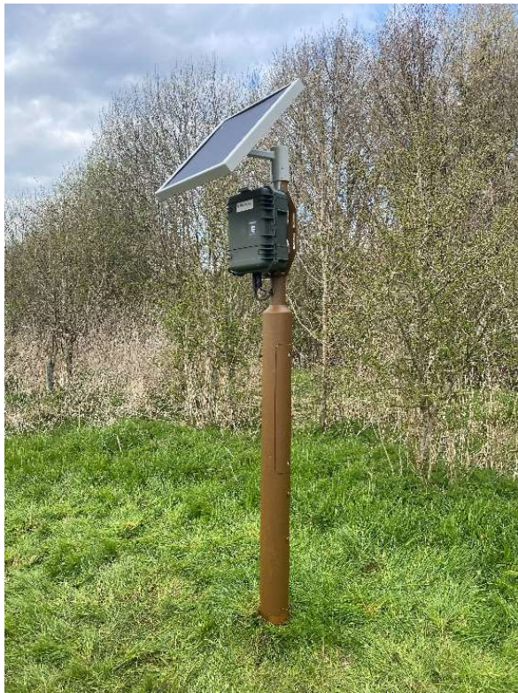
Solar/Telemetry Post Installation
