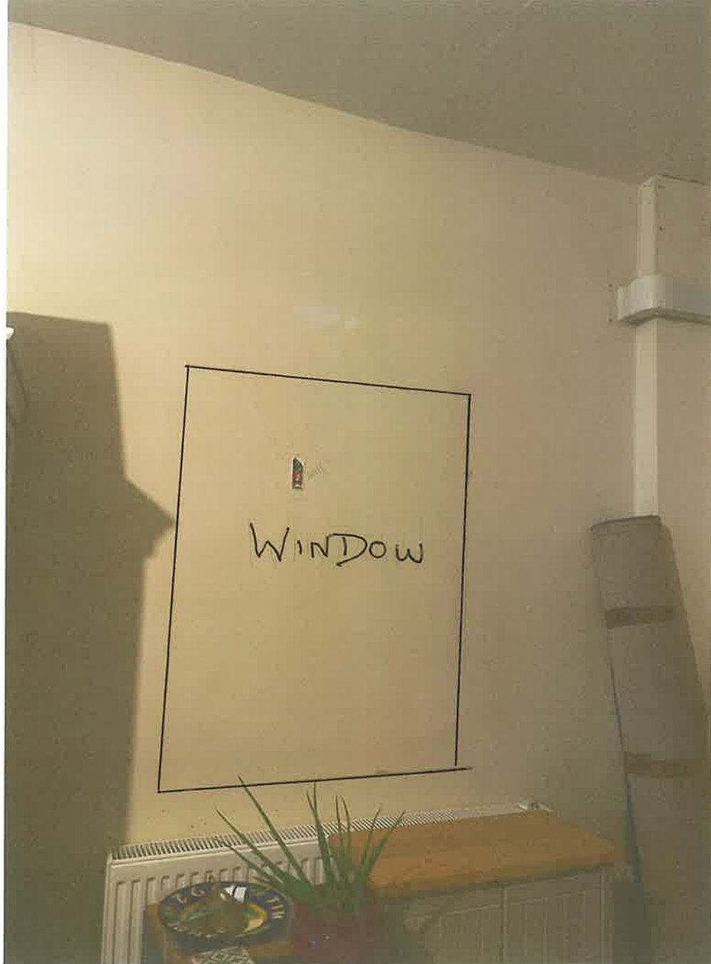
Photograph to show proposed window location within new lobby area.
