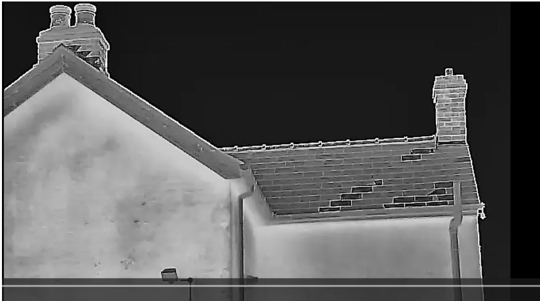
Plate 3: FoV from position 2 showing partially restricted view to eastern elevation
