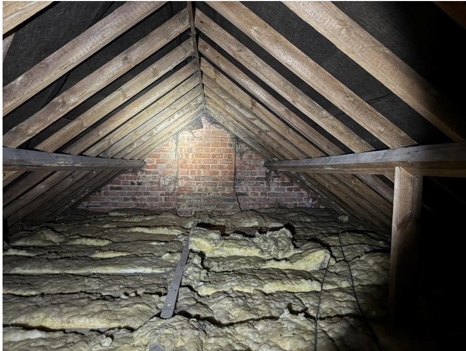
Plate A1: View towards northern gable
