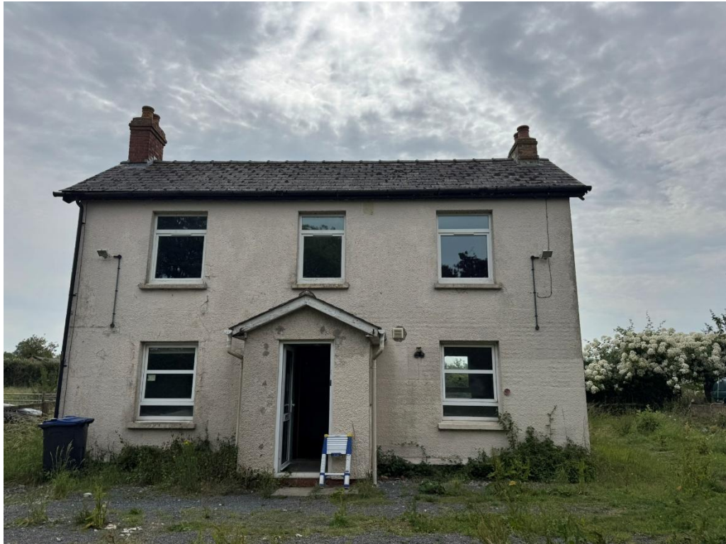
Plate 8: Front (western) elevation
