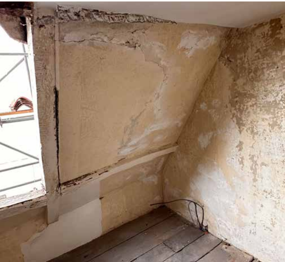
PHOTOS THIS PAGE: Above: Overtight spacing of laths - limited space for plaster to form ‘key’ Top right: Remaining lath and plaster ceiling in attic Bottom right: Indicative condition of sloped skelings
