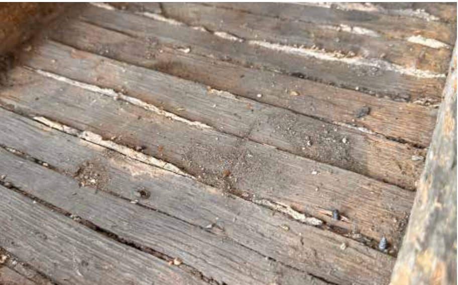
PHOTOS THIS PAGE: Above: Overtight spacing of laths - limited space for plaster to form ‘key’ Top right: Remaining lath and plaster ceiling in attic Bottom right: Indicative condition of sloped skelings
