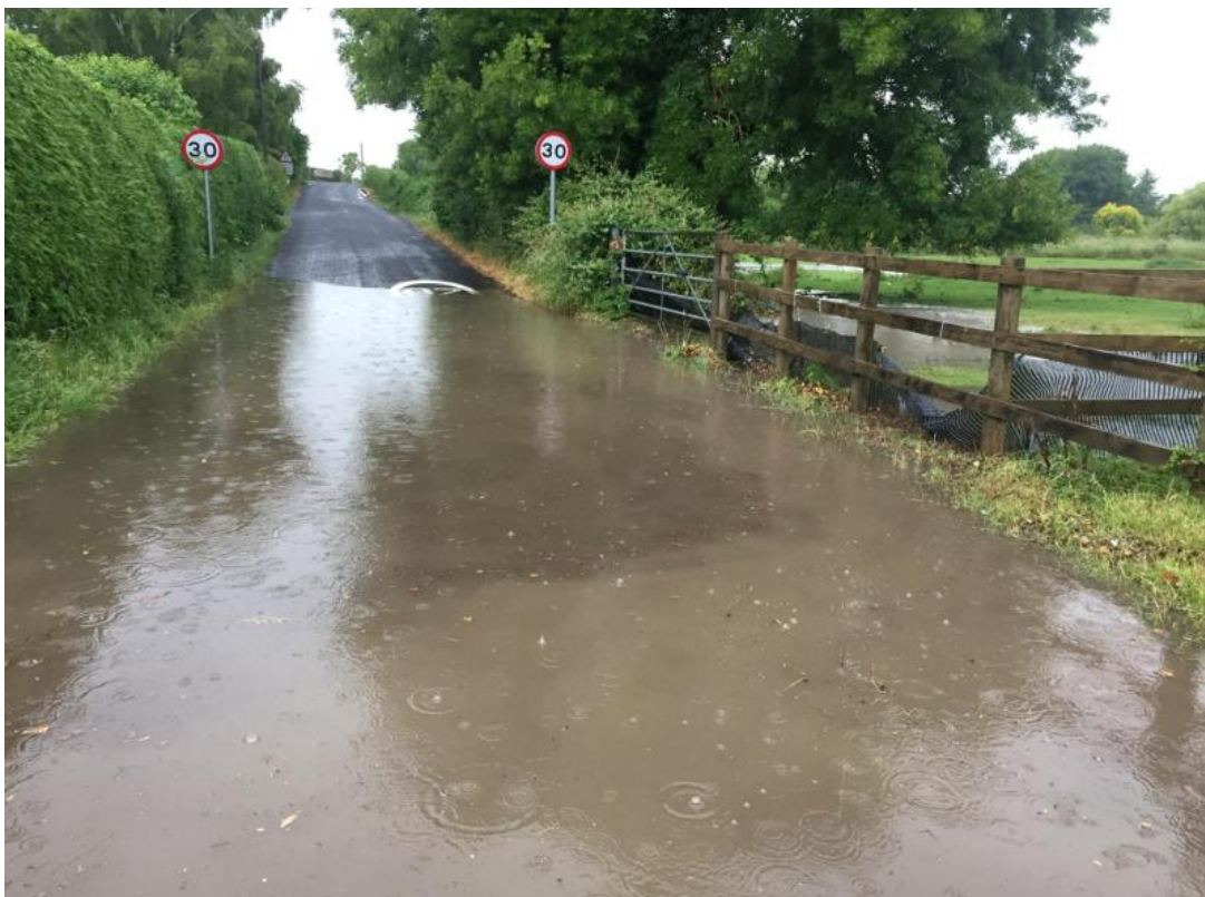
Photo 3-6b – Standing water on the road and in the paddock – June 2020
