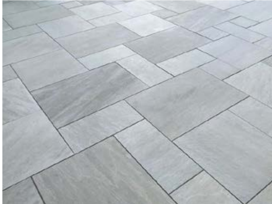
Natural stone paving, colour grey/ buff, sizes 300-600-900mm, or similar. For patio at the east of the house.
