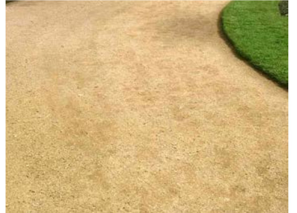
Self-binding gravel path. For use at rear and side of garage.
