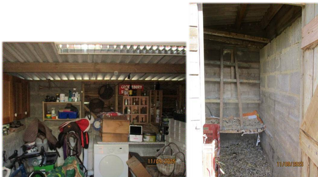
Interior rooms of Building 4 shed used for storage and chicken coop
