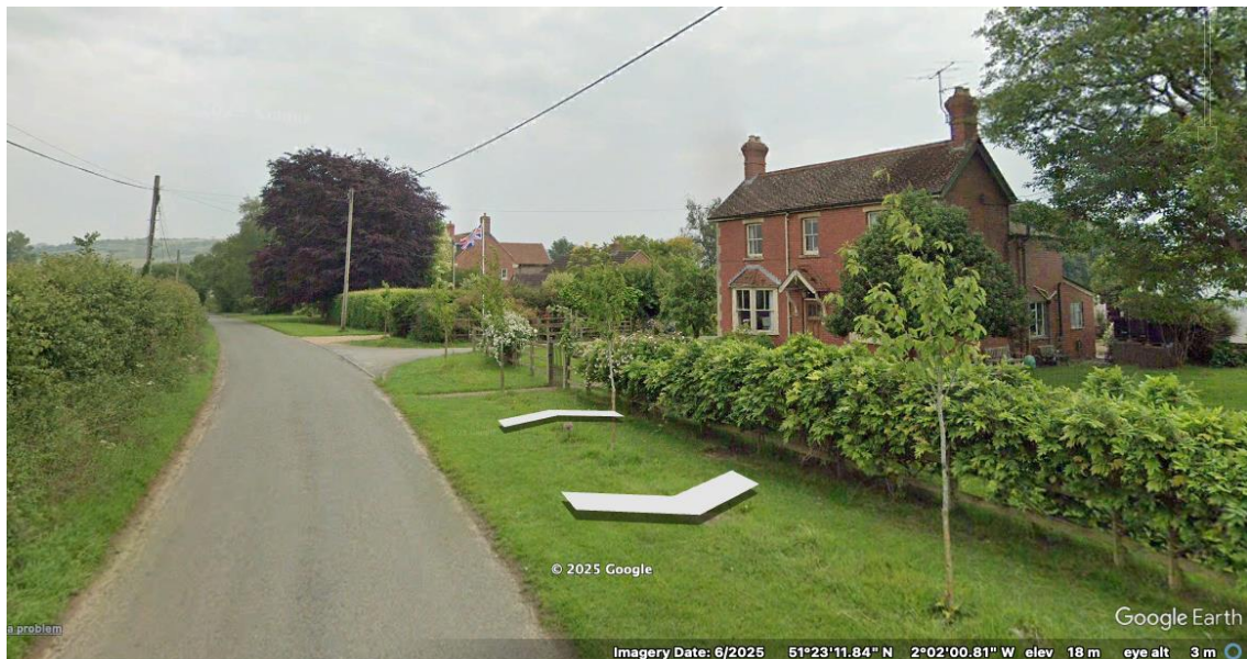
Figure 6 – 42 Yard Lane and neighbouring properties
