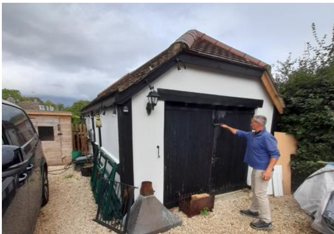
Fig. 34: View of the south-western end of the garage, looking north-east.
