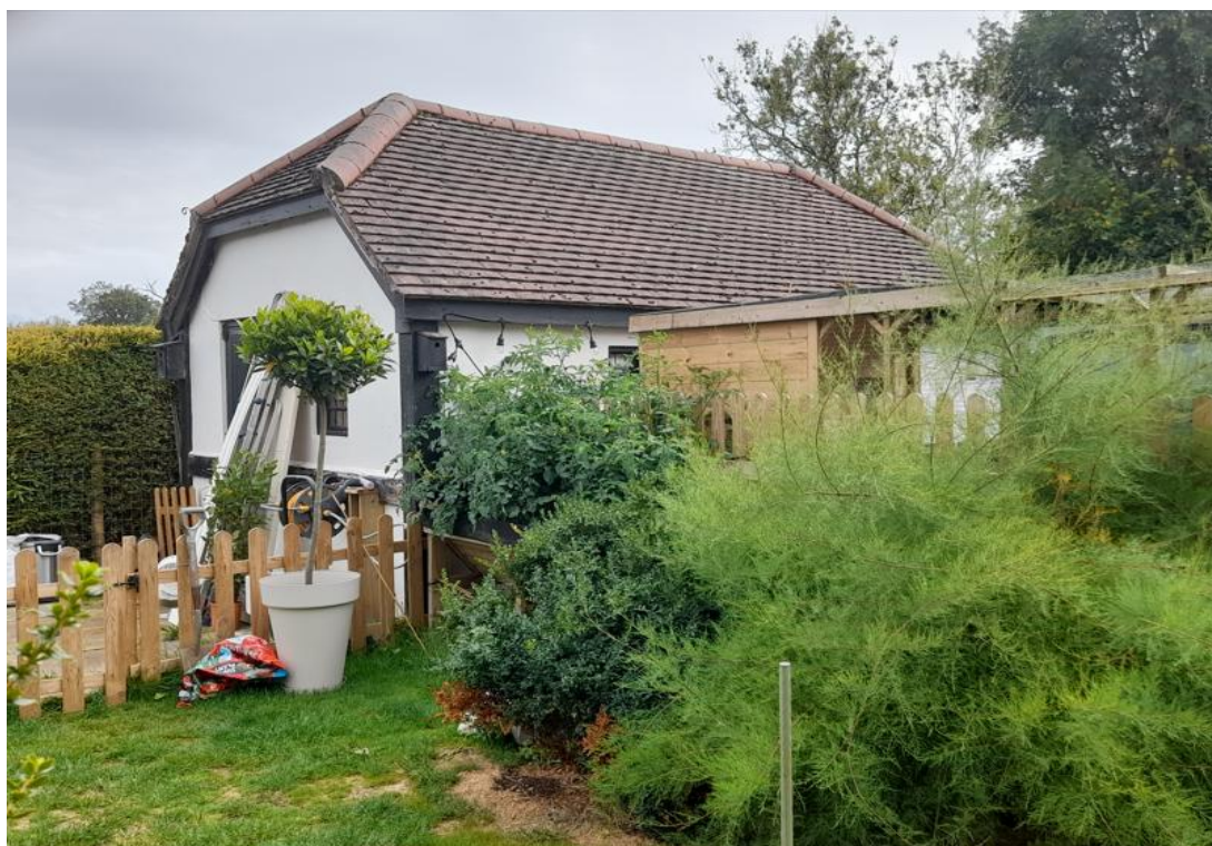
Fig. 33, View of the north-eastern end of the existing garage, looking west.
