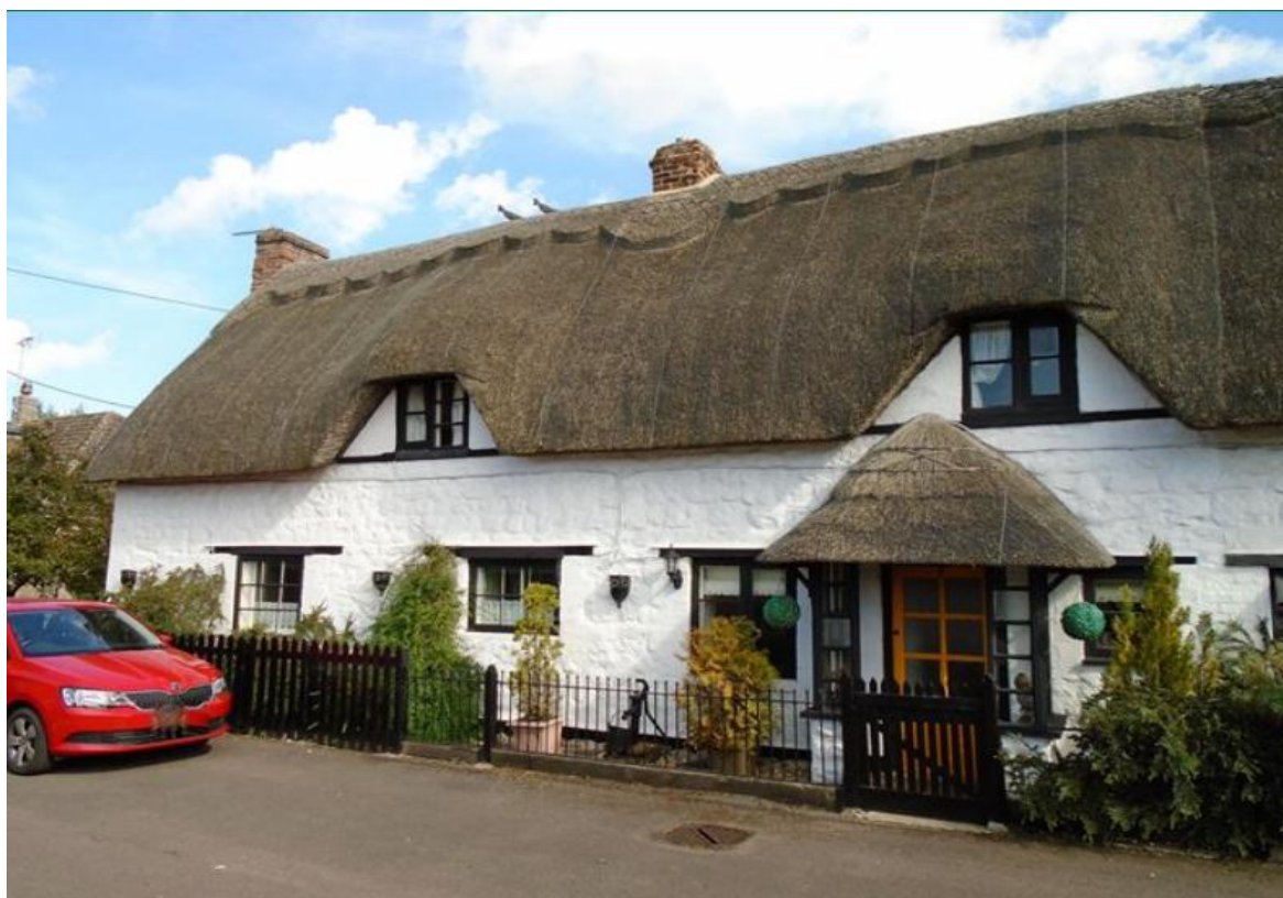
Fig. 5: View, looking east, of the south-west, front elevation of Nos. 5 and 6 Packhorse Lane (Historic England).
