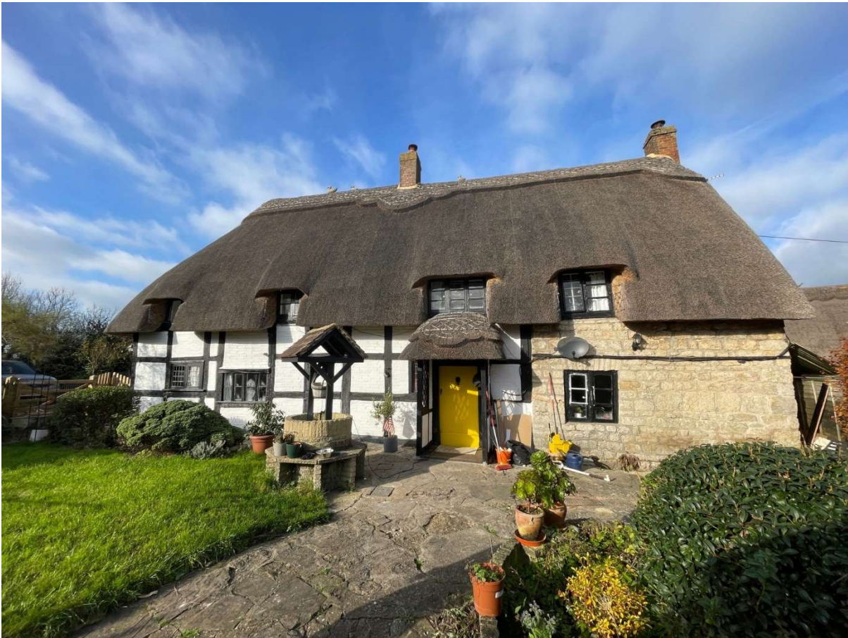
Fig 2.0 photograph of south east elevation
