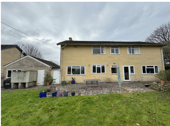
Photo of the existing rear elevation (North east facing)
