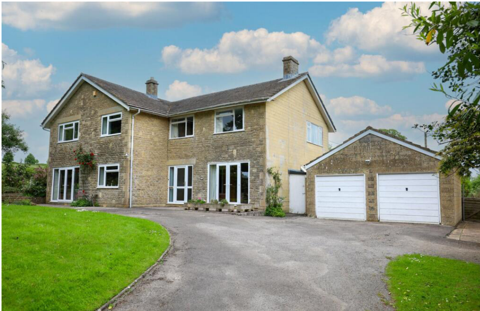
Photo of the existing front elevation (Southwest facing)
