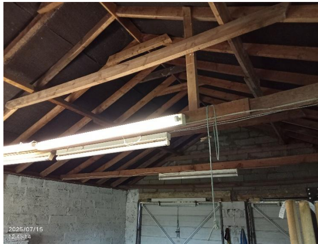
Photo 11: B2 internal roof.
