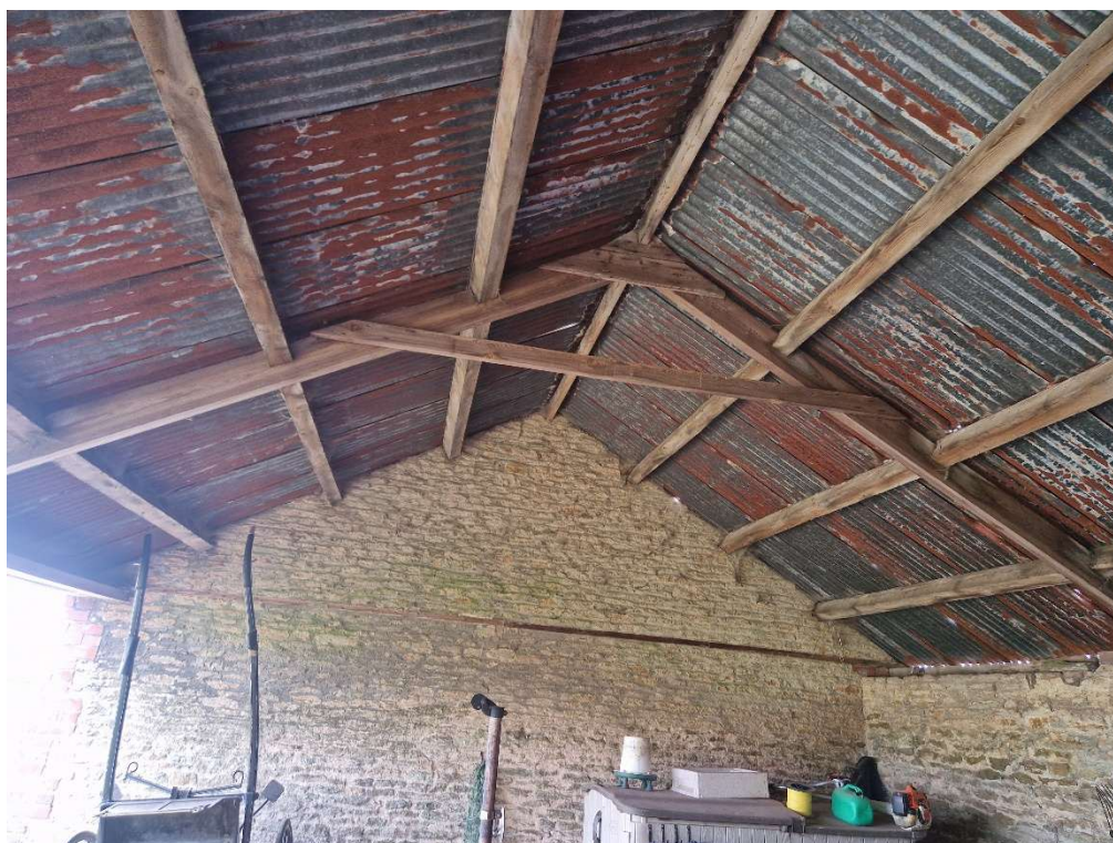
Internal view of barn
