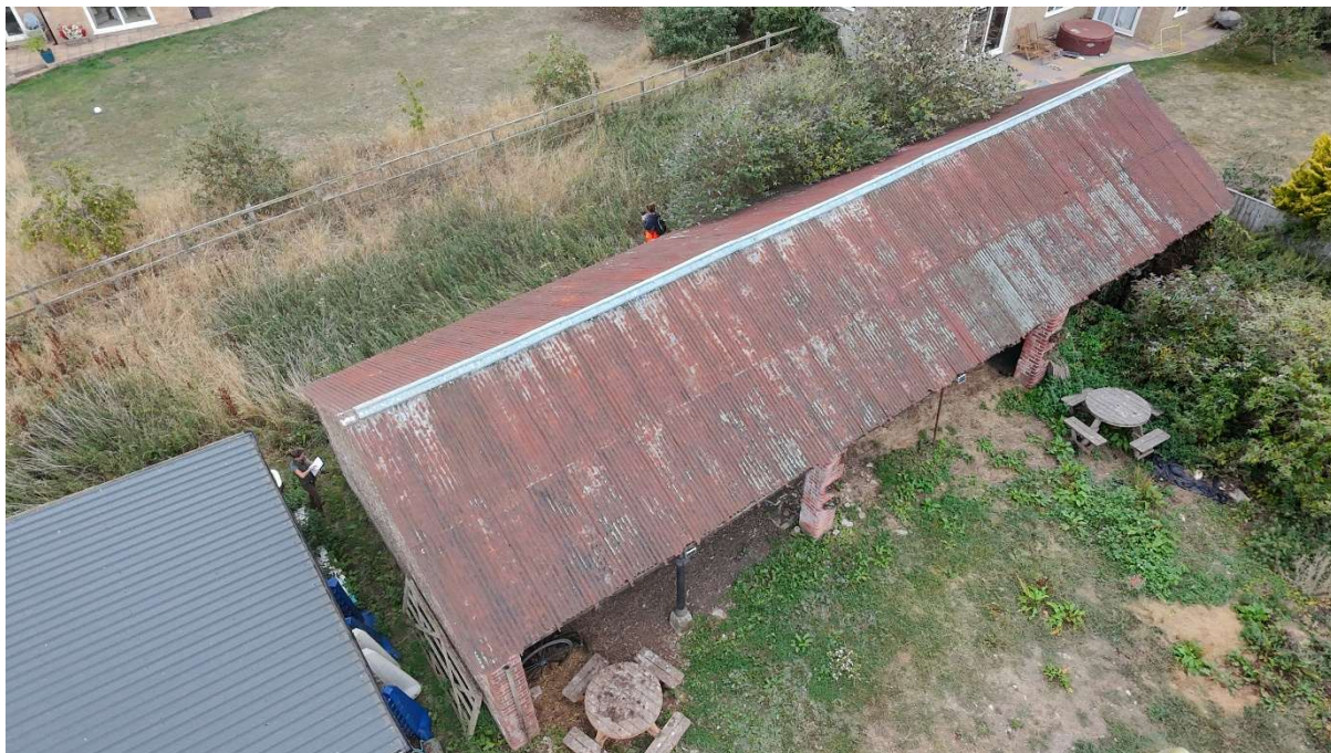
Aerial view of barn showing corrugated metal roof
