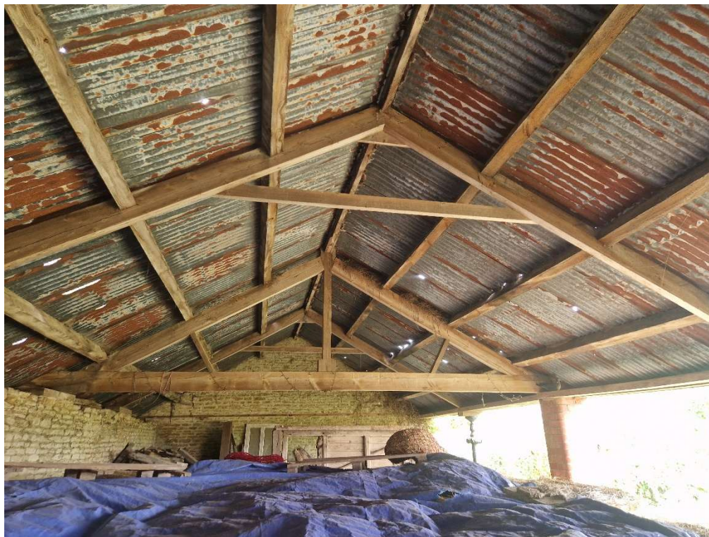
Internal view of barn
