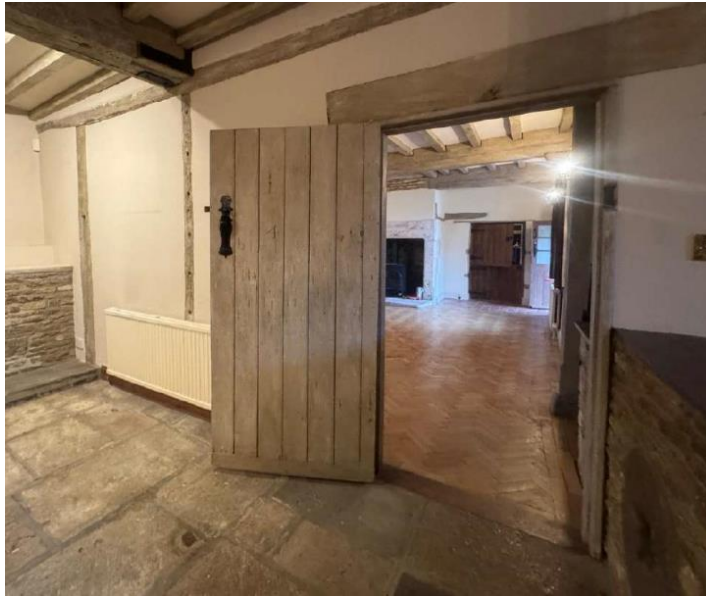
Photograph 3: During Refurbishment Work
