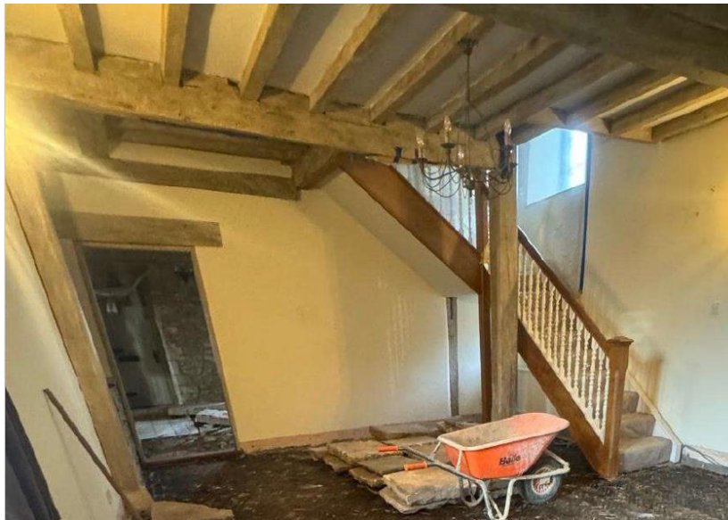
Photograph 1: During Refurbishment Work
