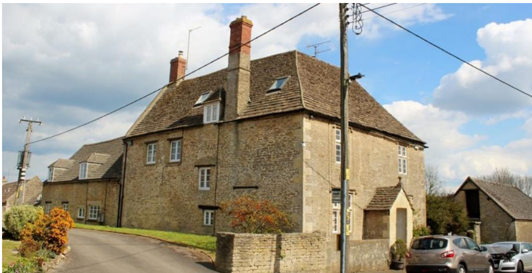
Photograph of Application Building (Source: Historic England Listing Webpage: 11 May 2021)
