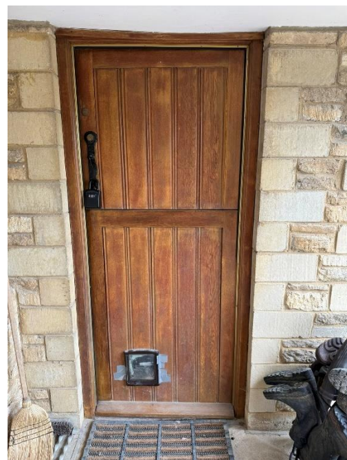
Existing Door No.2
