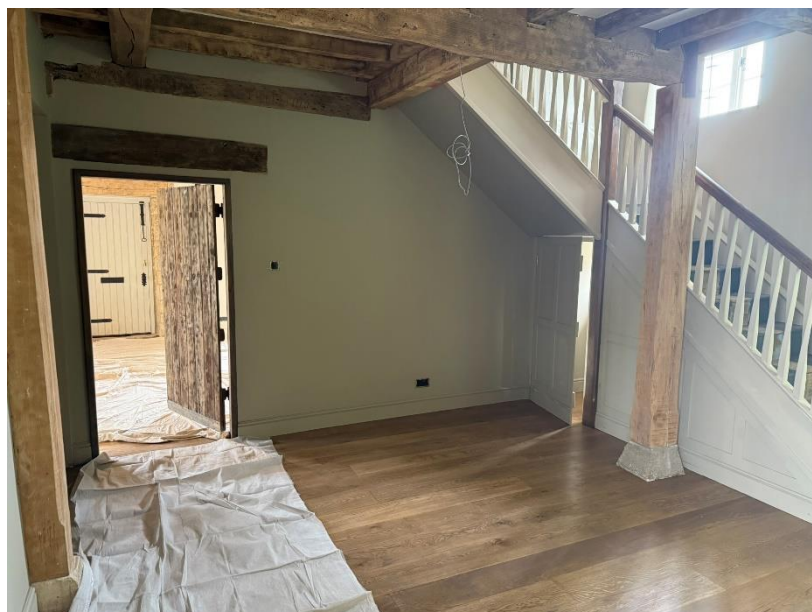
Photograph 2: Post Refurbishment Work
