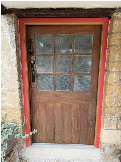
Existing Door No.1
