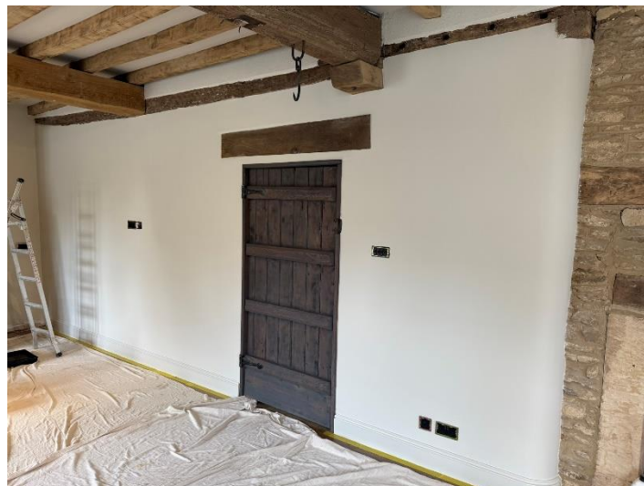
Photograph 4: Post Refurbishment Work
