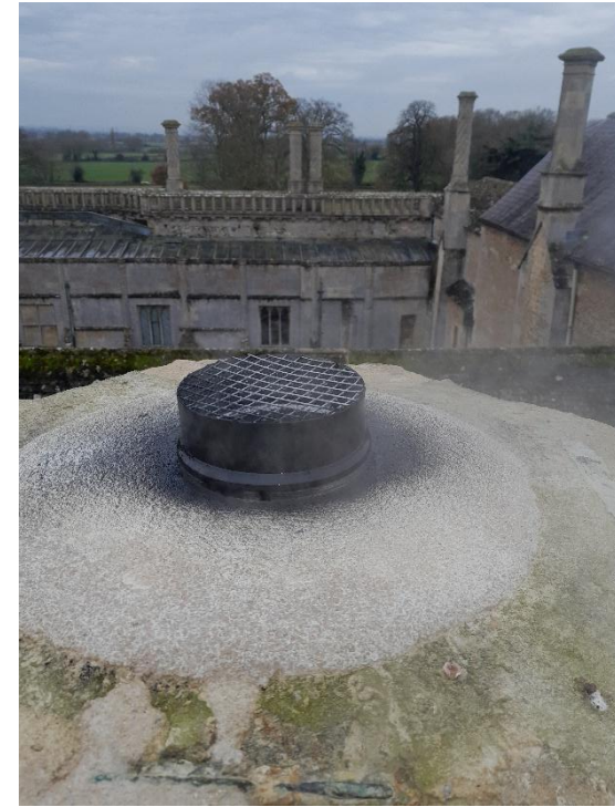
Photos 5-7 showing the dismantled chimney capping, the works underway and the completed terminal with finished flaunching.
