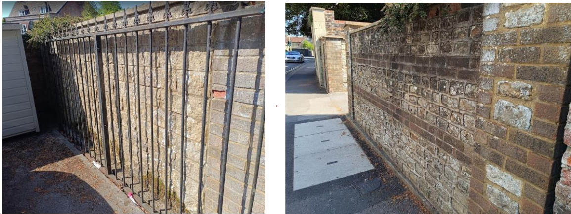
Figure 6: Rear facing (LHS image) and front facing (RHS image) elevations of wall
