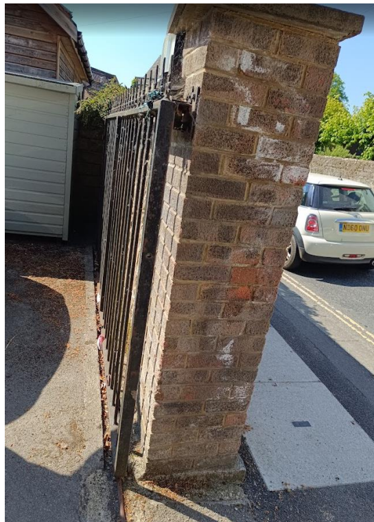
Figure 7: Stone capped modern gate pier on southern side of existing vehicular entrance point to site
